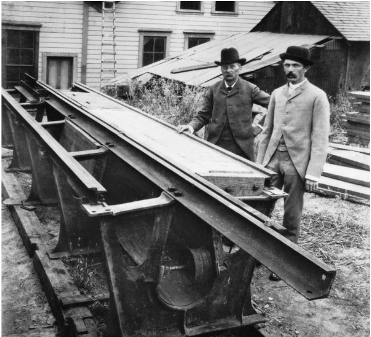
Frederick Wood and John Fowler of the Temple Street Cable Railway pose with a sample piece of cable car railway roadbed. Courtesy of the Title Insurance and Trust, and C.C. Pierce Photography Collection, USC Libraries.
