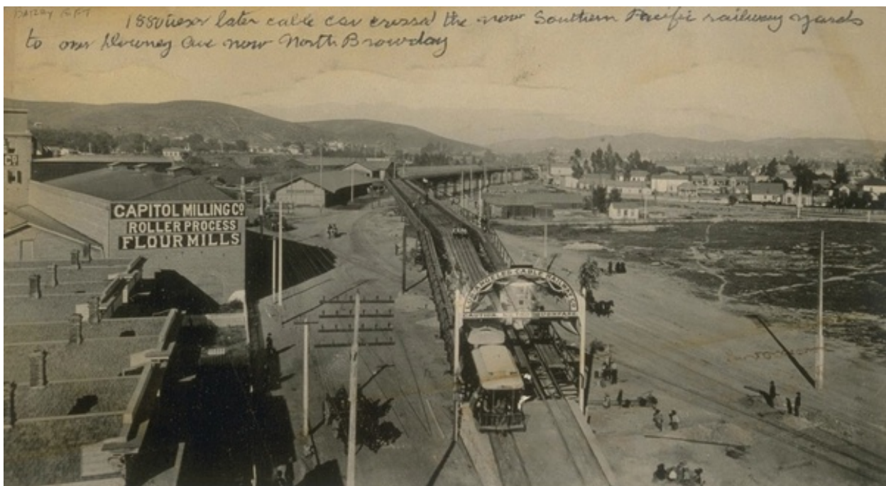
A soaring viaduct carried the Los Angeles Cable Railway's tracks over the Southern Pacific railyard and Los Angeles River on their way to East Los Angeles (today, Lincoln Heights). Courtesy of the William C. Barry Collection of Los Angeles Area Photographs, Bancroft Library, UC Berkeley.
