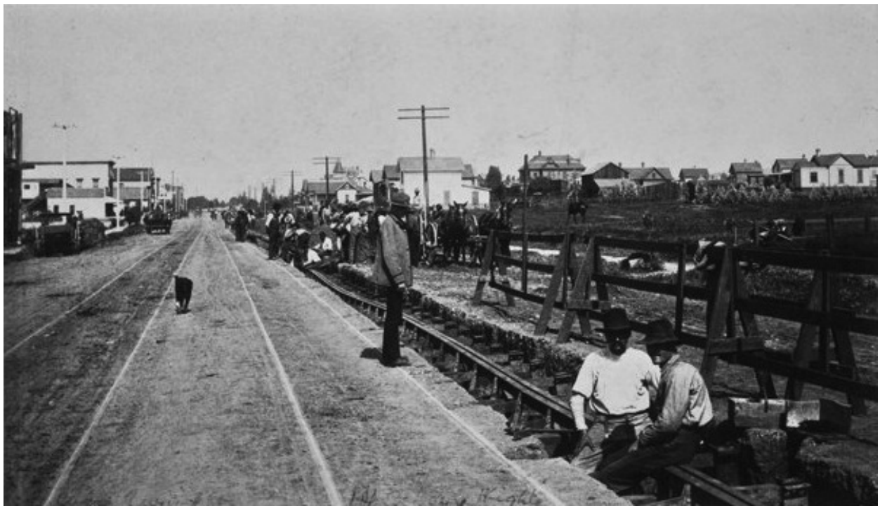
Workers installing cable car tracks in Boyle Heights. The tracks to the left were used by horse-drawn streetcars, which cable cars replaced. Courtesy of the Metro Transportation Library and Archive.
