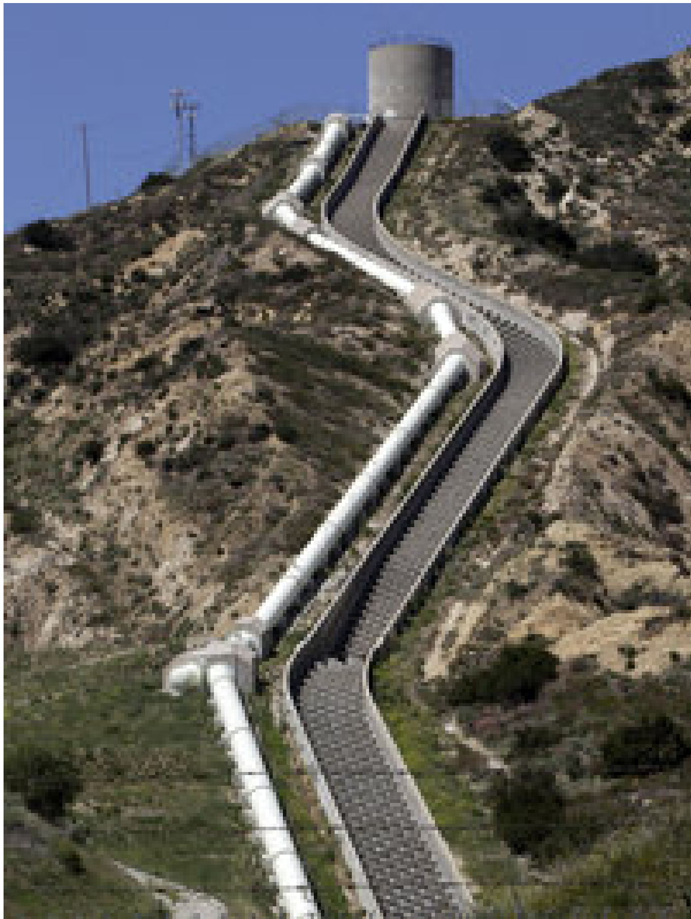
Water flows through The Los Angeles Aqueduct Cascades near Newhall Pass in Sylmar, Calif. The aqueduct, which carries millions of gallons of water to the city of Los Angeles, turns 100 years old this week.
