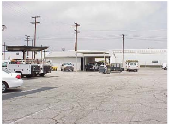
Non-Revenue Repair Area
