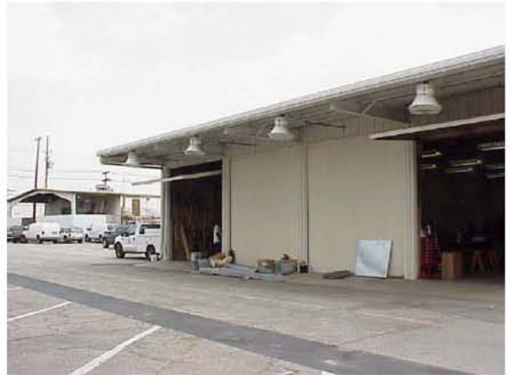
Facilities Maintenance, Rail Shop
