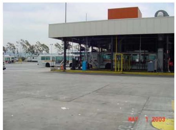
Maintenance Fuel Island
