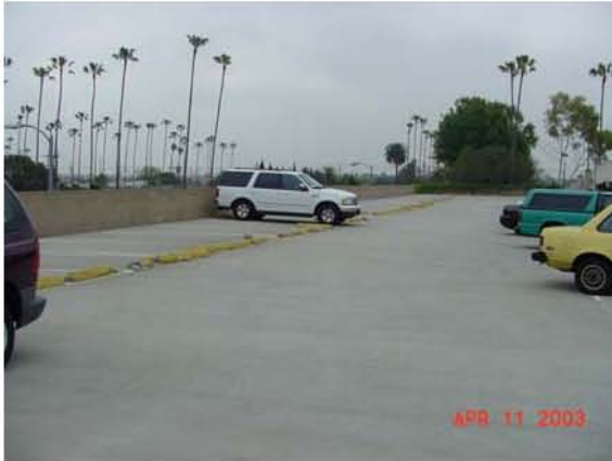
Restricted Roof Parking
