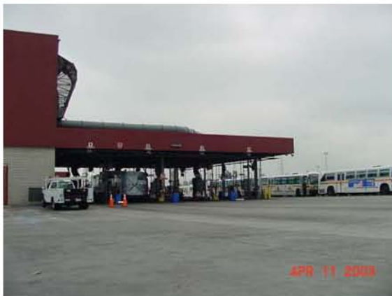
Main Yard at Fuel Island
