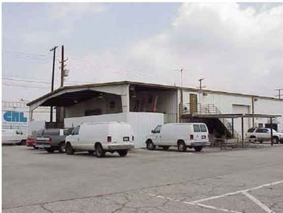
Fare Box Building
