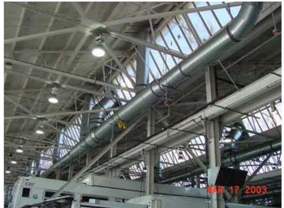
Maintenance Building -Interior
