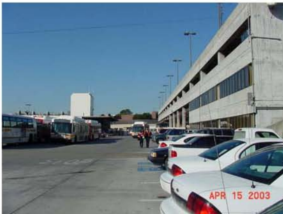
Yard, Looking West
