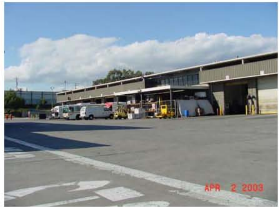
Maintenance Building, South End
