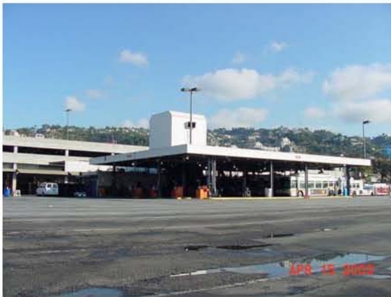
Main Yard, Fuel Island Northward
