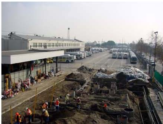
Underground Tank Replacement
