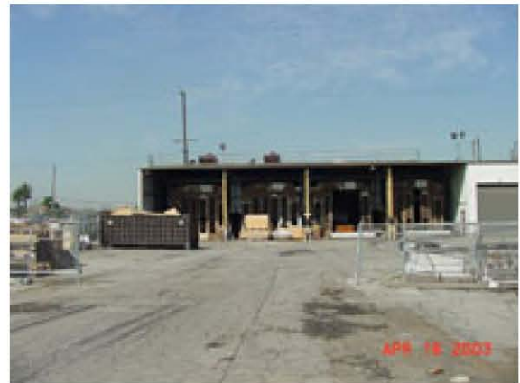
Rear of Property, Westside
