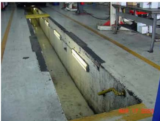
Maintenance Building – Inspection Pit
