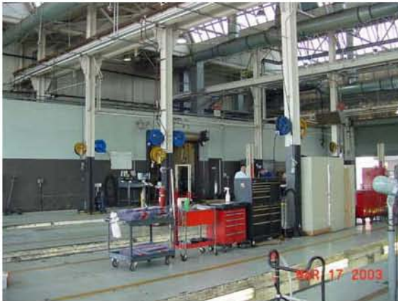
Maintenance Building – Interior
