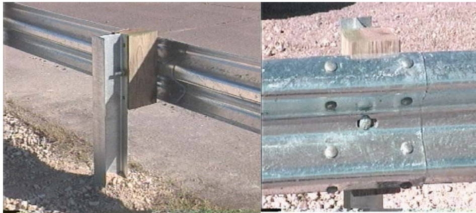
Figure C6-1: Modified G4(1S) guardrail with routed wood blockouts
