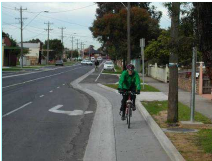
Figure 3.11 Kerbed cycle lane with parking (in background of picture), Melbourne, Australia (H Barber)
