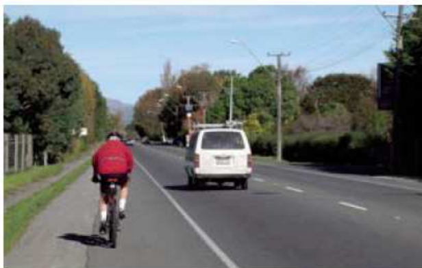
Figure 3.2 A wide sealed shoulder on Marshland Rd, Christchurch, New Zealand (LTNZ 2005, p38)
