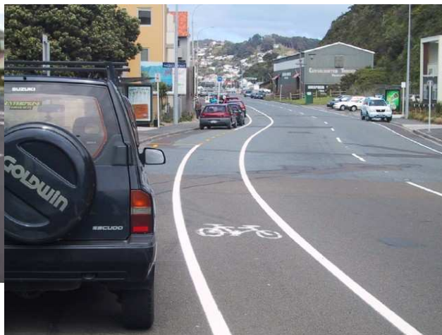
Figure 3.9 Cycle lane with solid white line next to parked cars, Wellington, New Zealand (unknown source)
