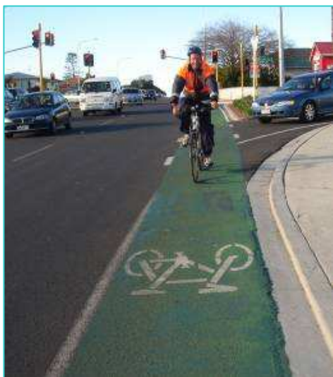
Figure 3.10 Painted cycle lane, New Zealand (North Shore City Council)
