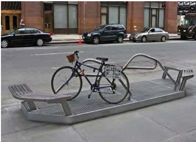
Figure 4-3 Raised Ventilation Grates
