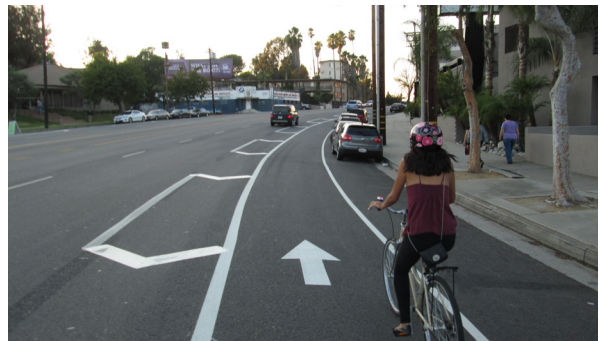
Class II Buffered Bicycle Lane (Dedicated On-Street)
