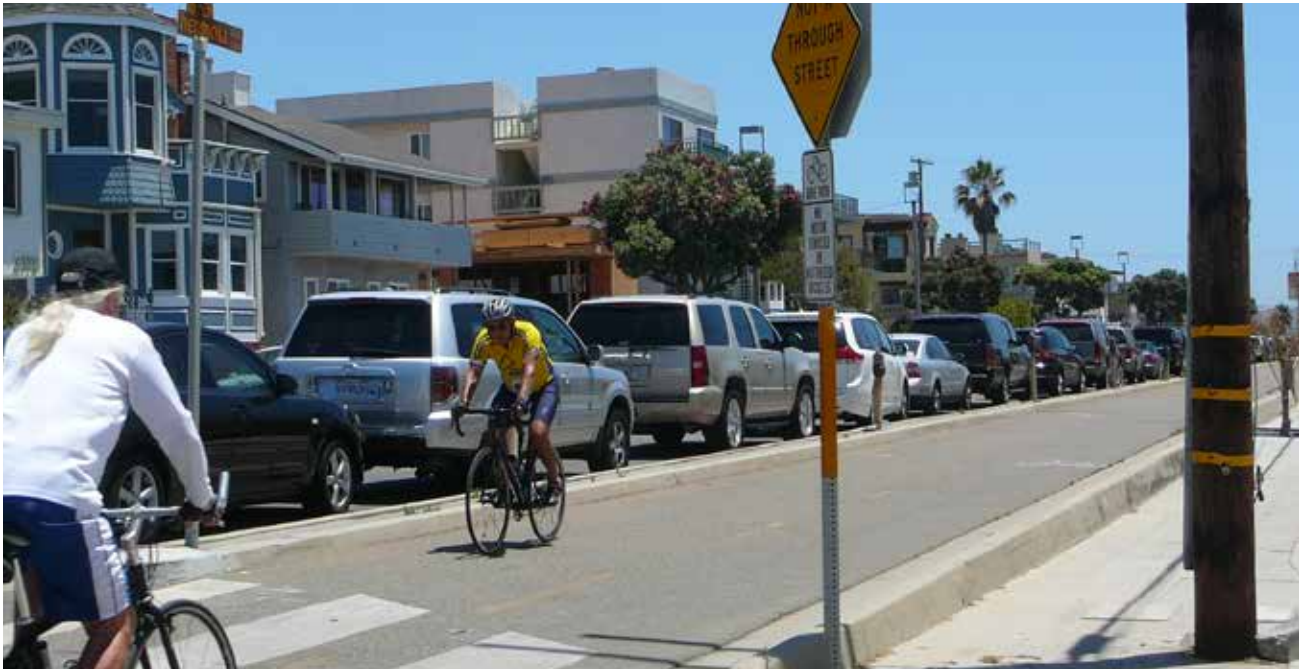
Hermosa Beach, CA - A two-way protected bicycle lane provides a safe, separated space for users of all ages and abilities.
