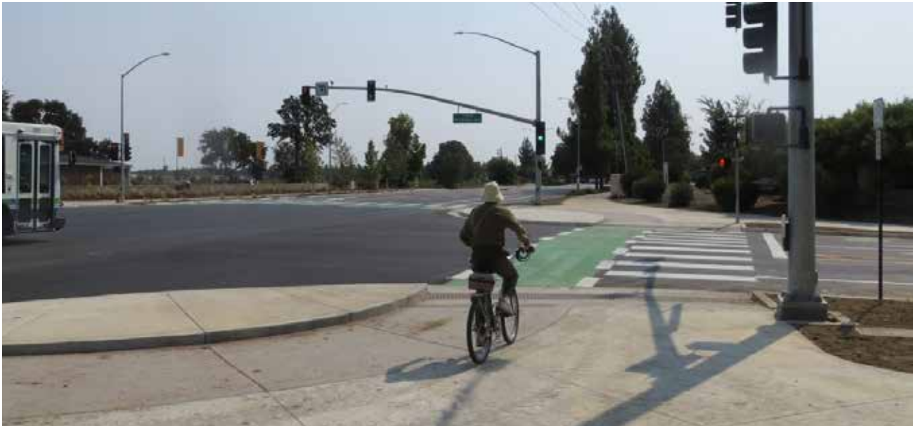
Davis, CA - The protected intersection connects buffered bicycle lanes and conventional bicycle lanes.
