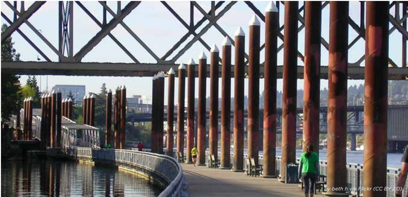
Portland, OR - a floating path fills a gap in the Eastside Esplanade shared use path corridor.
