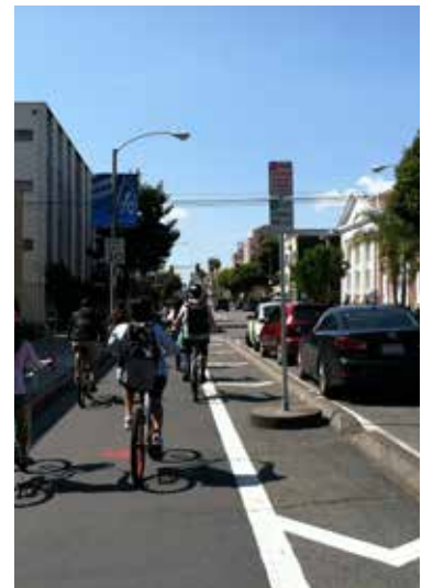
Long Beach, CA - Protected bicycle lanes can combine various physical separation methods, such as parking stops, flexible bollards, planters and motor vehicle parking.
