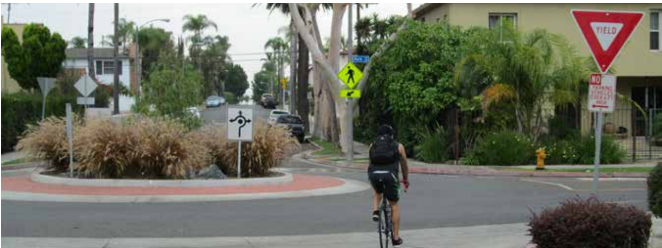
Long Beach, CA - Bicycle boulevards use speed and volume management techniques to create comfortable conditions for bicycling in mixed traffic. Alternating parking creates a chicane to slow traffic speeds.
