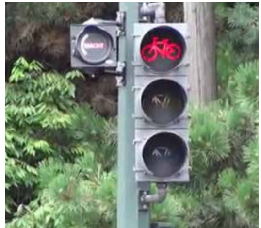
Portland, OR - A countdown signal beside the bicycle signal head informs waiting bicyclists of the timing remaining until a green signal.
