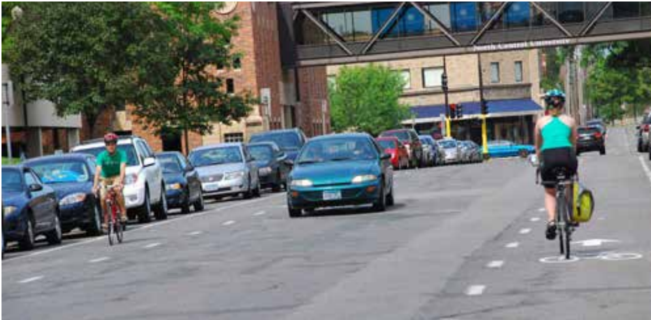
Minneapolis, MN - This downtown street is too narrow for both conventional bicycle lanes and parking. Advisory bicycle lanes allow the road to continue to serve parking and motor vehicle access, while providing a prioritized space for people to ride.
