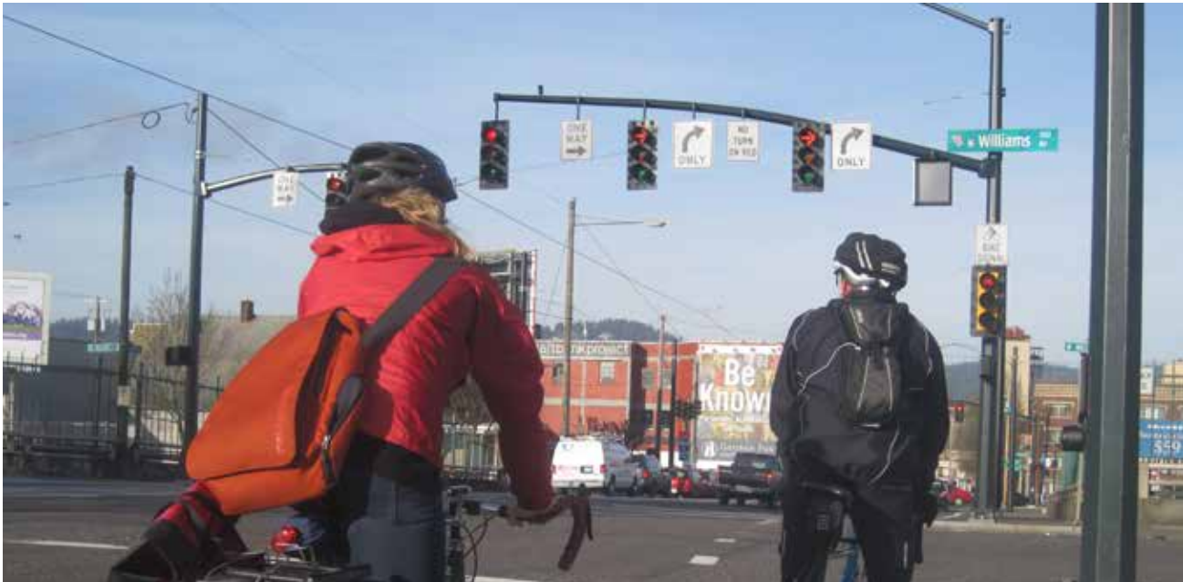
Portland, OR - A bike lane adjacent to double right turn lanes normally requires a stressful, difficult maneuver to avoid conflict. With a bicycle signal, conflict is regulated and the conditions are improved.
