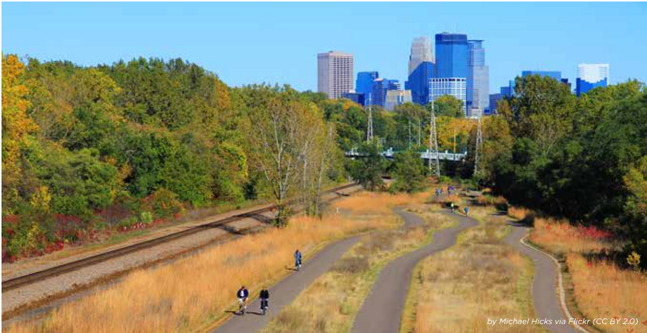
Minneapolis, MN - The Cedar Lake Trail offers tread separation by mode and direction.
