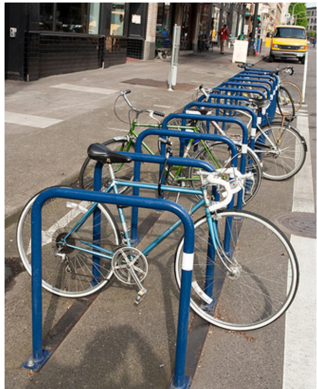
On-street bicycle corrals can secure 12 or more bicycles within a typical curbside parking space.
