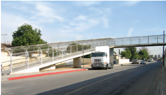
Pedestrian Bridge over I-5 Fwy (north end)
