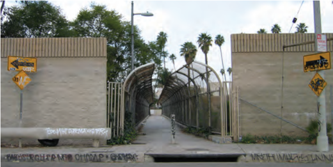
Estudillo at Ped Bridge (facing south)
