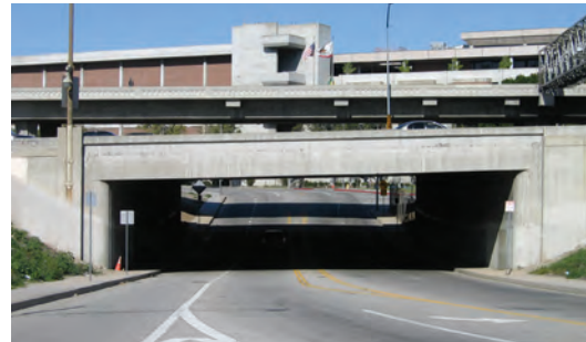
Center at 101 Fwy underpass (facing north)
