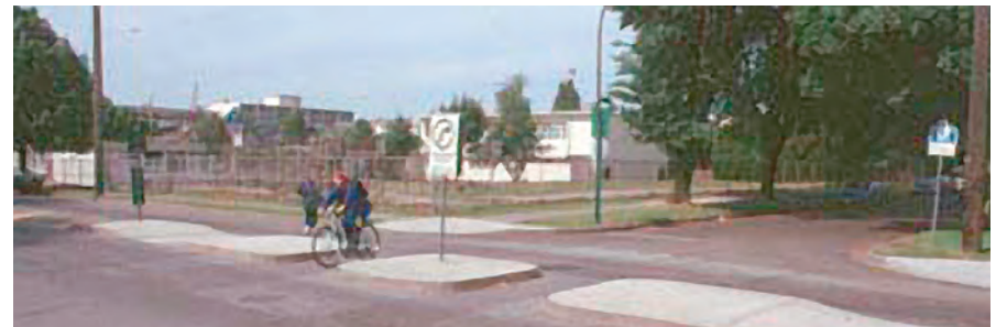
Median Refuge / Crossing Island (location unknown) Source: Pedestrian and Bicyclist Information Center (PBIC)
