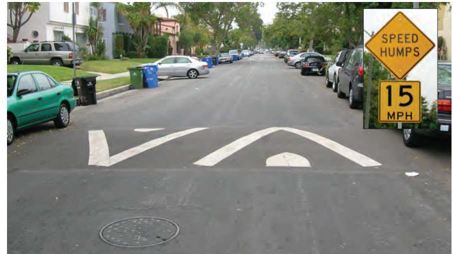
Typical speed hump, Los Angeles Source: LACBC
