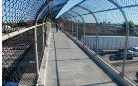
Existing Ped Bridge over I-5 at Eastman Avenue accommodate bicyclists.
