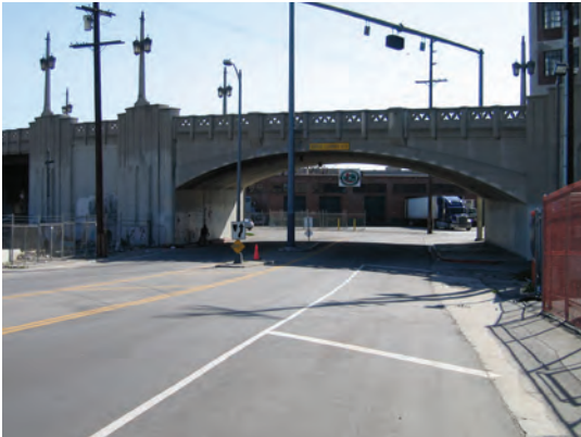
Santa Fe at 4th St Bridge (facing south)
