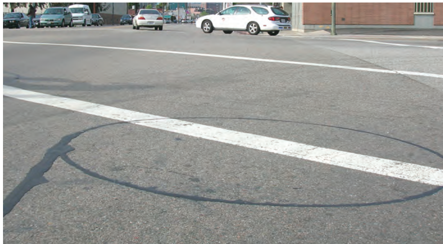
Typical circular traffic signal actuator, Los Angeles (6th & Central) Source: LACBC
