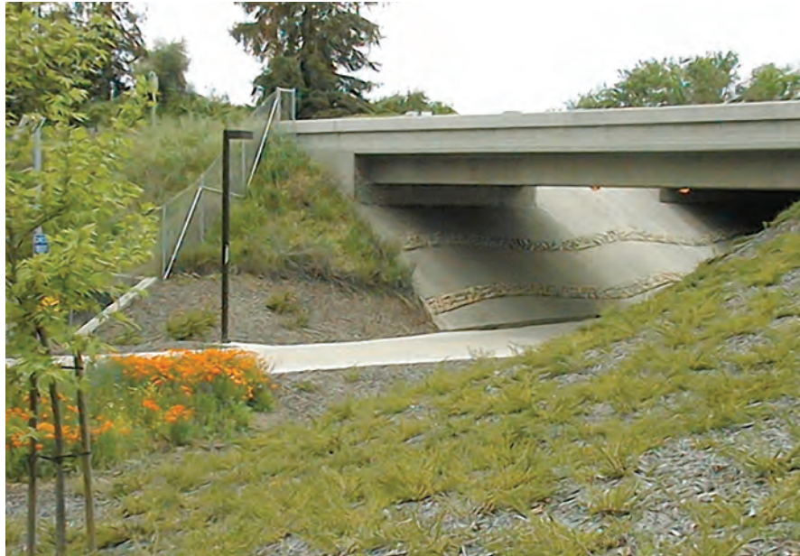
I-80 Freeway Undercrossing: Davis, CA
