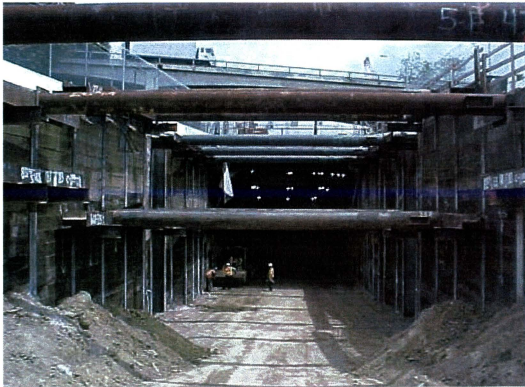
Gold Line Eastside Extension – West Portal entrance Gold Line Eastside Extension – excavation of utility trench under US 101
