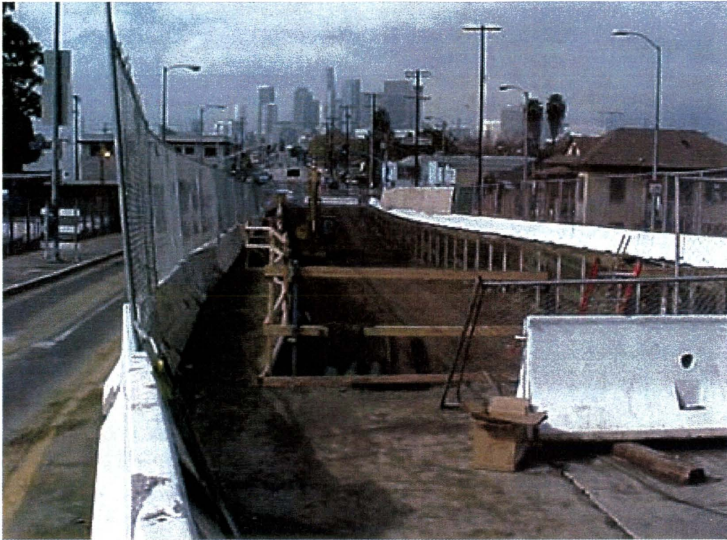
Gold Line Eastside Extension – West Portal excavation
