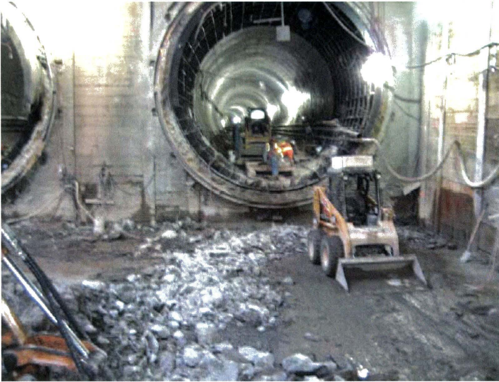
Gold Line Eastside Extension Project – West End of Soto Station
