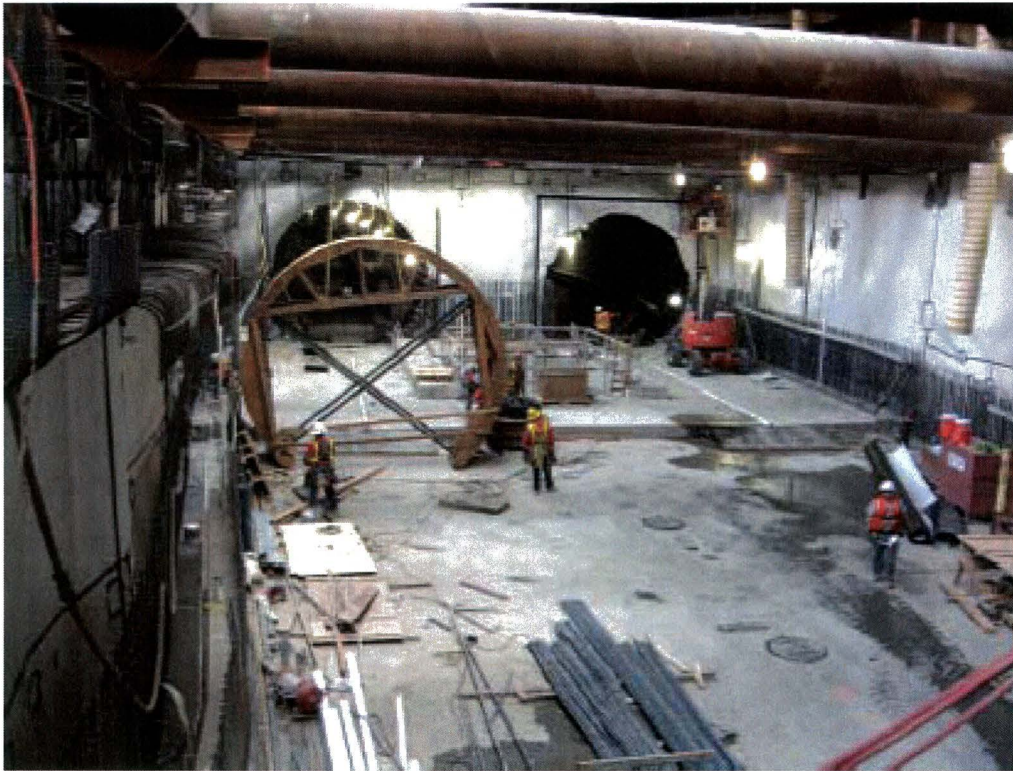
Gold Line Eastside Extension Project – Construction at Soto Station
