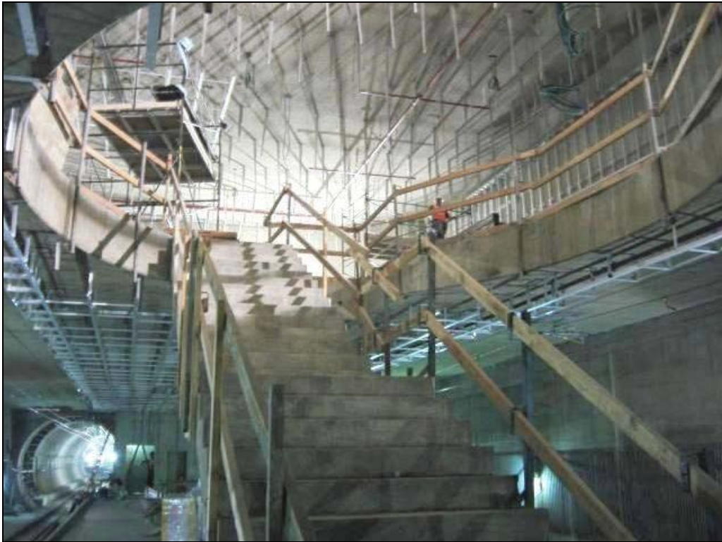
Soto Station – Stairs from Platform
