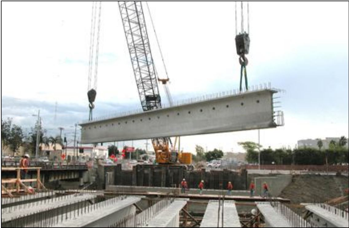
Installation of Girders for National Bridge
