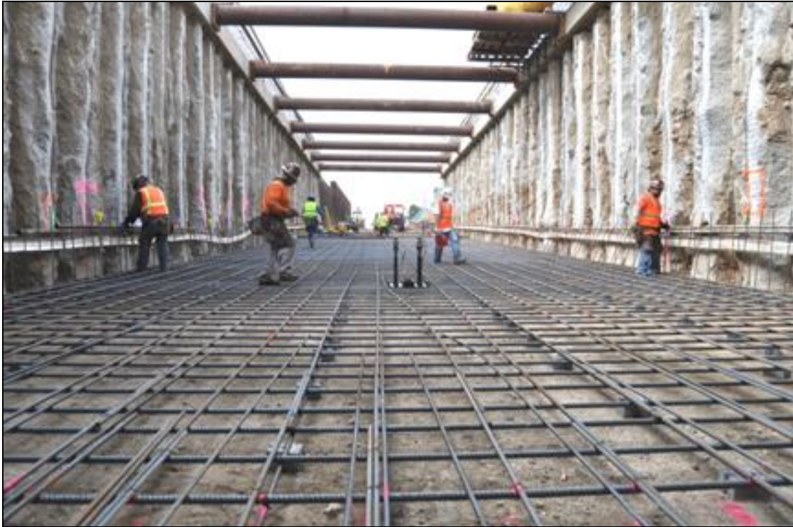
Rebar Work on Trench Slab
