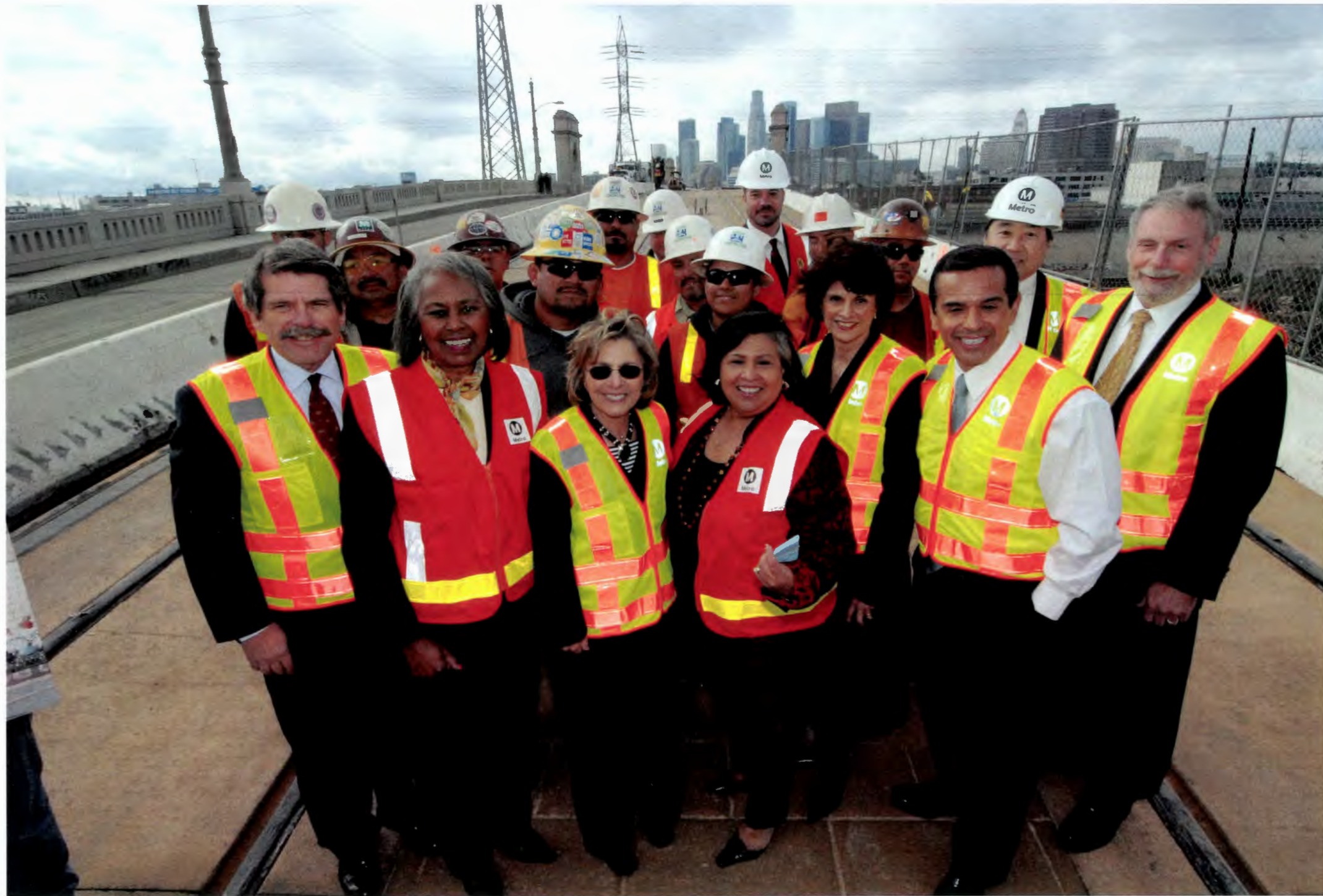
aFebruary 20, 2008: U.S. Senator Barbara Boxer, U.S. Representative Lucille Roybal-Allerd and Metro officials inspect the construction site of Eastside Extension.
