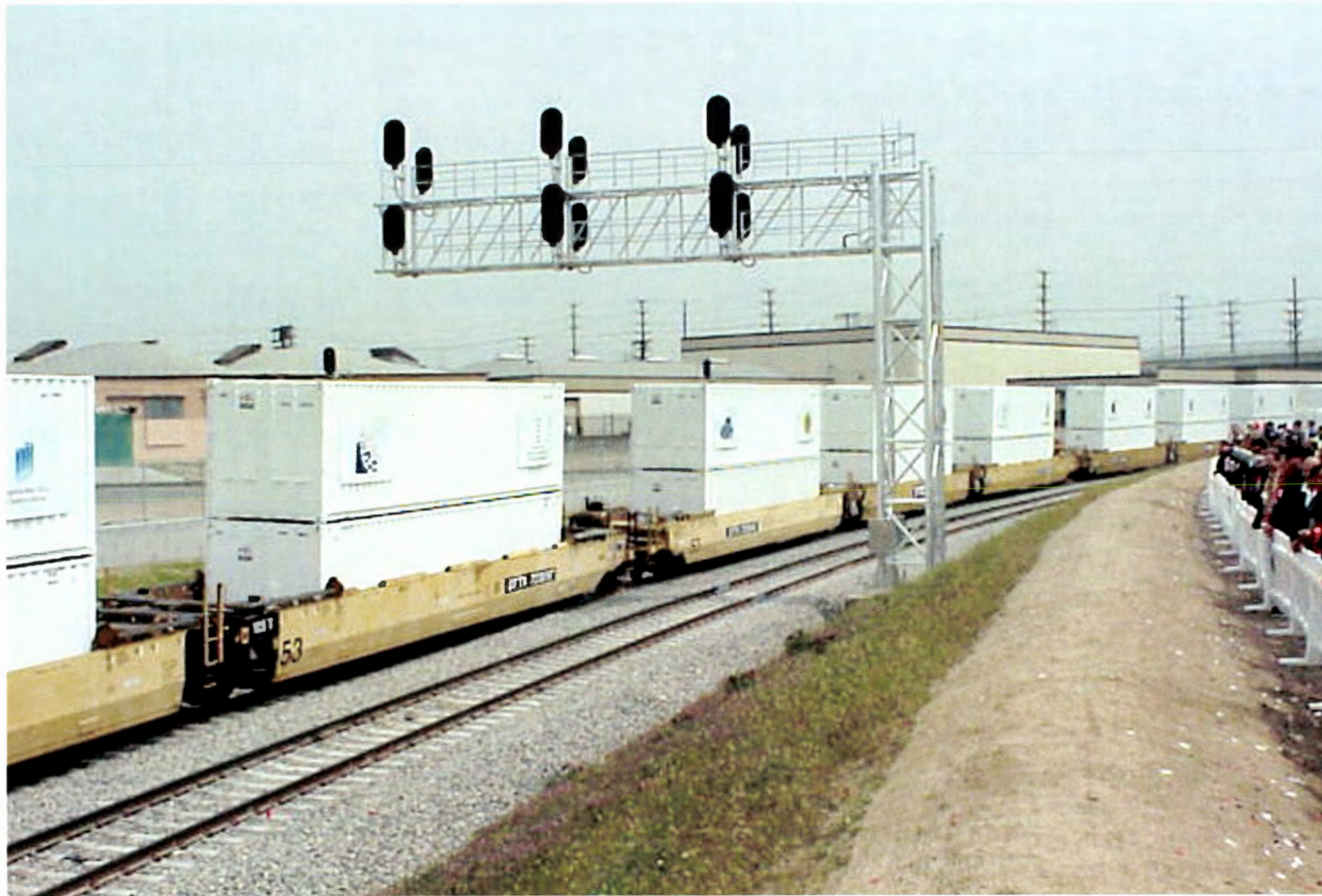
Alameda Corridor Dedication April 12, 2002.
