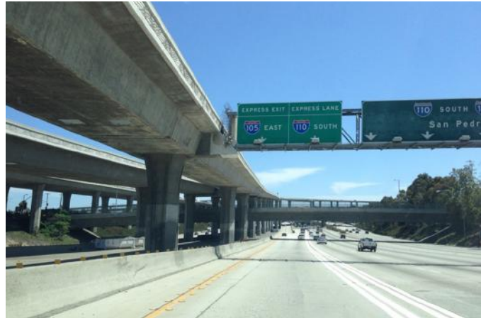
Figure 13: Photo of Existing I-110/I-105 HOV/HOT Direct Connectors
