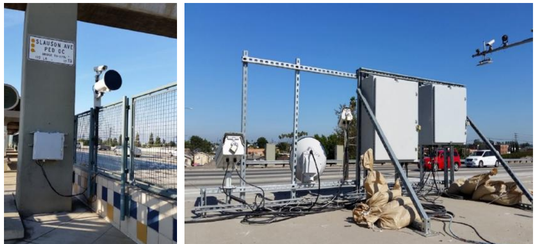
Figure 18: VPDS Camera and Equipment
