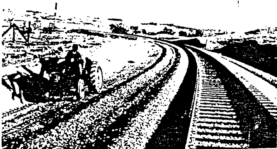
New track serves coal mine in Wyoming. Tractor operator seeds banks along right of way.
