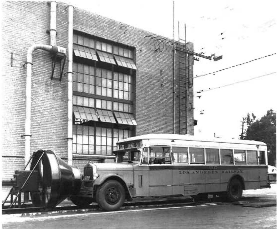
Figure 13. LARy was very proud of this bus dynamometer, taking many photos of the installation. This view from the 1930s shows clearly the west window arrangement, which was filled in during the 1982 remodeling 25
