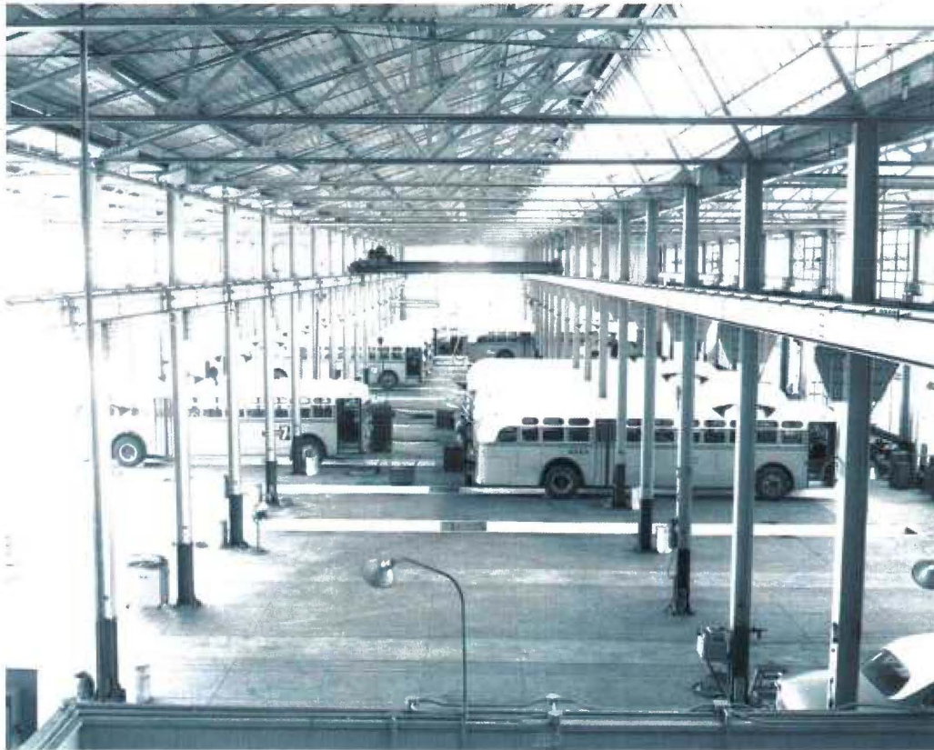
Figure 12. Inside the bus repair garage in the 1950s, showing how little modified it was from new; it remains largely unchanged today 24
