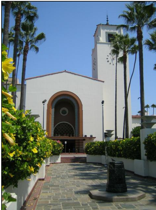
Figure 39 – Current photo of exterior front of Union Station showing main entrance and clock tower. Photo by Holly Kane.
