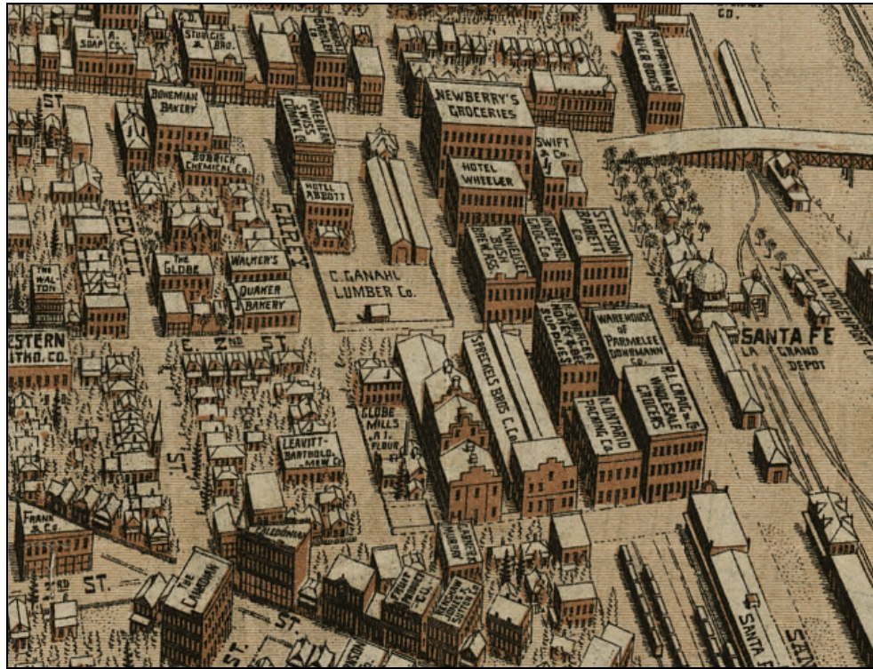
Figure 21 – Detail from 1909 bird’s eye map showing Santa Fe’s La Grande station and the surrounding neighborhood. The First Street viaduct over the Los Angeles River is shown in the upper right corner. Library of Congress, American Memory Project.
