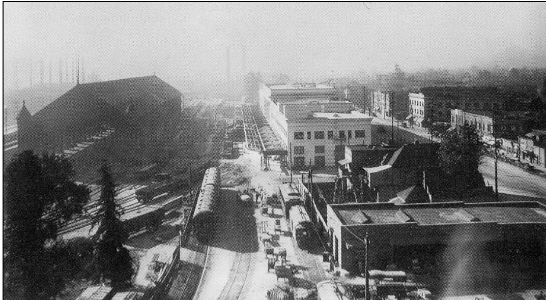
Figure 13 – Construction underway of new Central Depot (white building to right) next to the Arcade Depot train shed remnants (dark structure on left).
