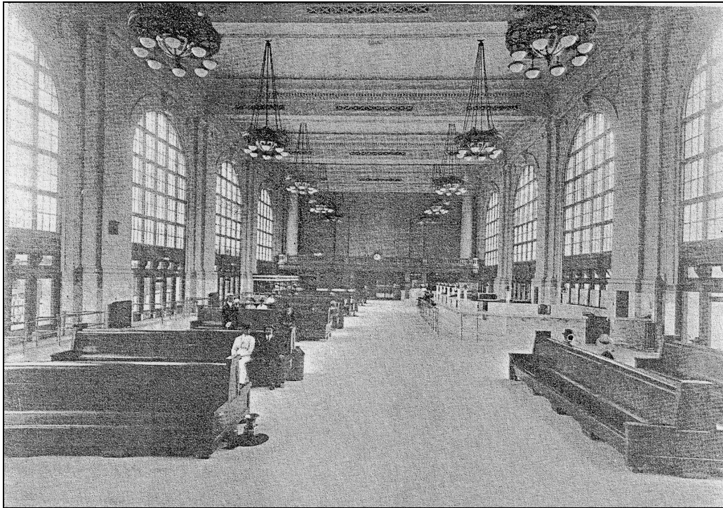
Figure 16 – General waiting room at Central Depot. Architects: Parkinson & Bergstrom. Originally published in The Architect and Engineer , February 1917.
