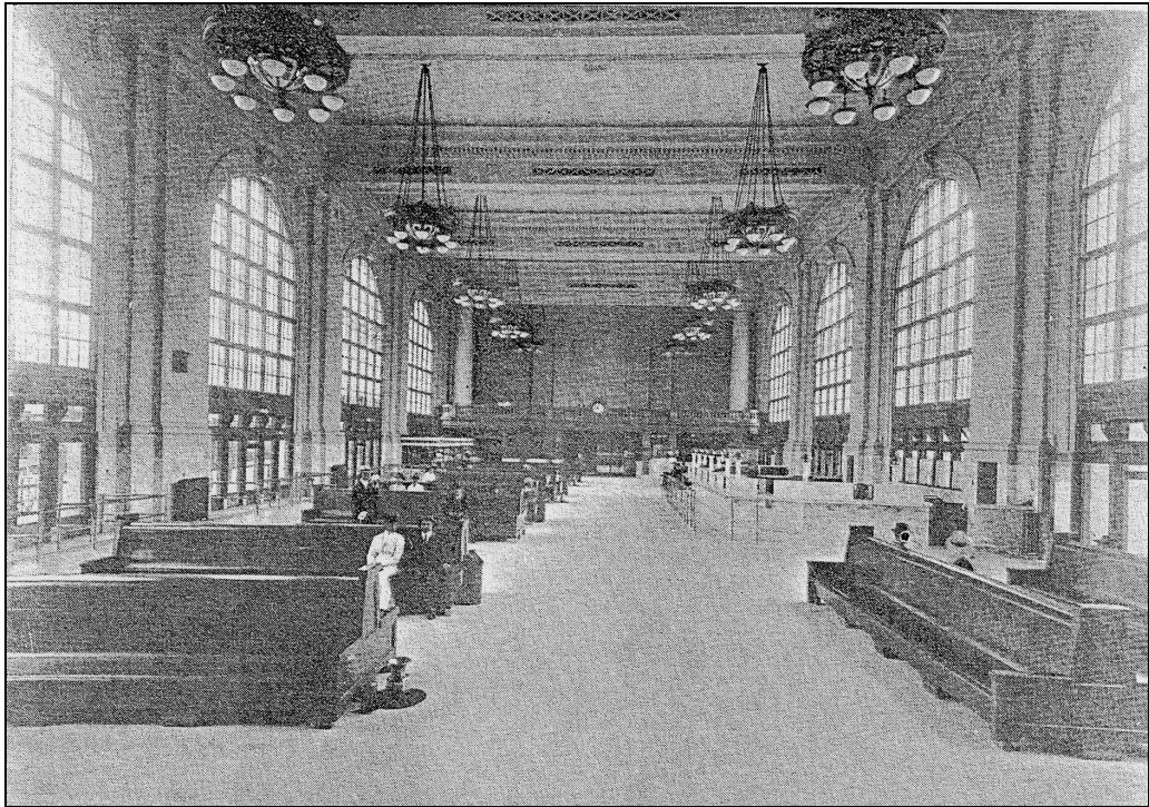
Figure 16 – General waiting room at Central Depot. Architects: Parkinson & Bergstrom. Originally published in The Architect and Engineer , February 1917.
