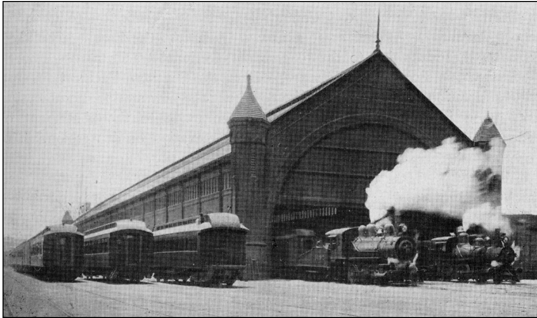
Figure 10 – Southern Pacific's Arcade Station train shed.
