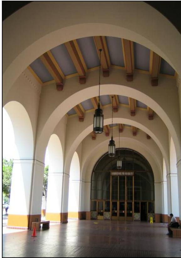
Figure 40 – Current view of arcaded walkway between the former Harvey House restaurant and the vestibule. Photo by Holly Kane.
