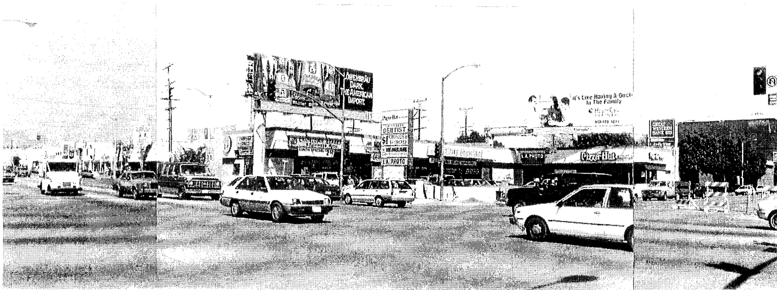
Figure 4-5.4: Looking northeast from the corner of Whittier and Atlantic Boulevards.
