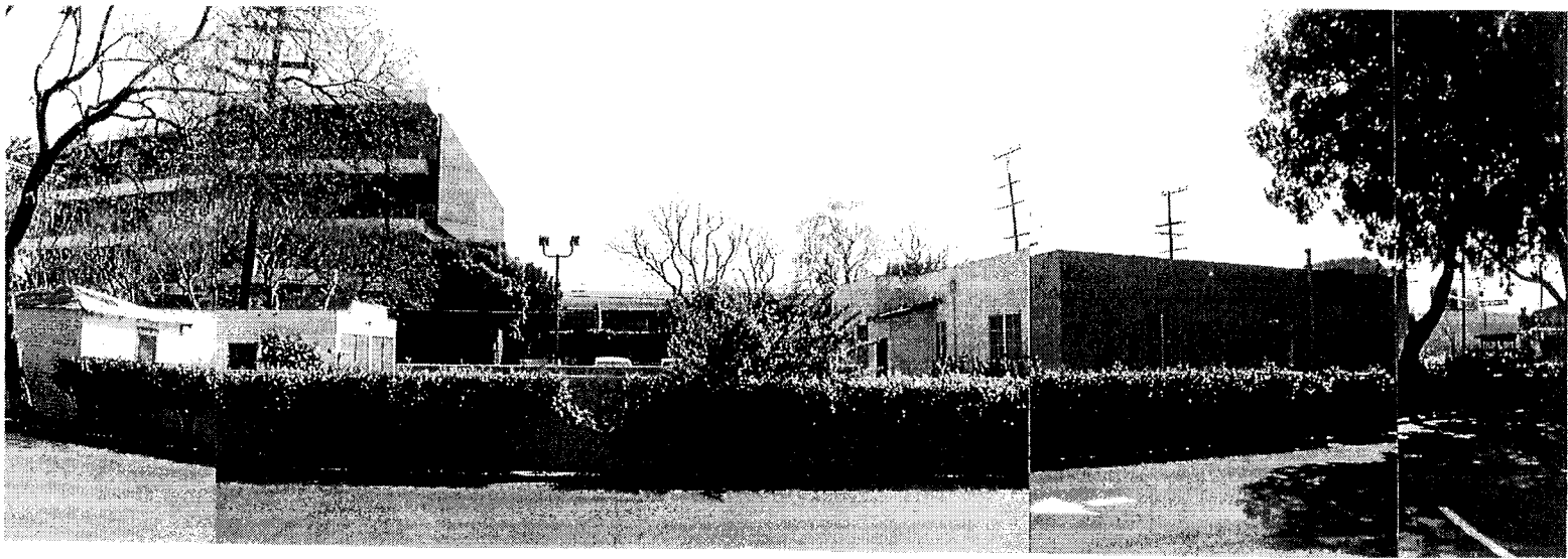
Figure 4-5.5: View of proposed site looking south from the north wall adjacent to the southern edge of residential properties north of the site.
