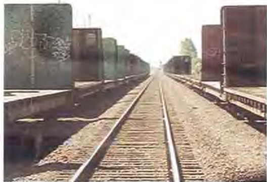
Siding 2– City of Torrance (M.P. 23.3)
