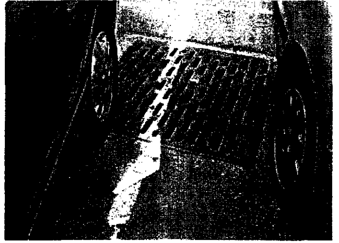
5. A view of the typical drain located on the southern portion of the Site.
