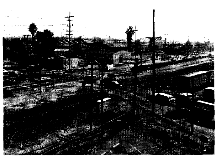
PHOTO 4: Doran Street at San Fernando Road
