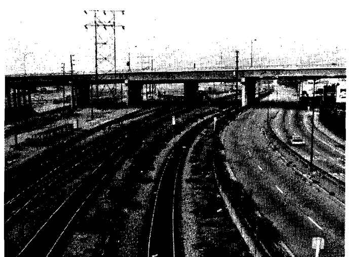
PHOTO 6: Rail alignment near Riverside Drive.
