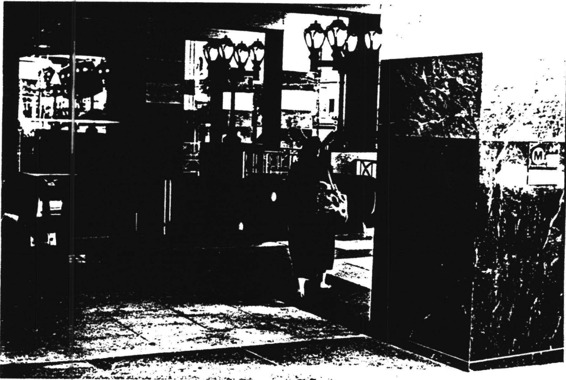
Plate 5.3 An example of how a subway portal can be made part of the adjacent building design. (This is the Metro Center/7th Street station in downtown Los Angeles.)
