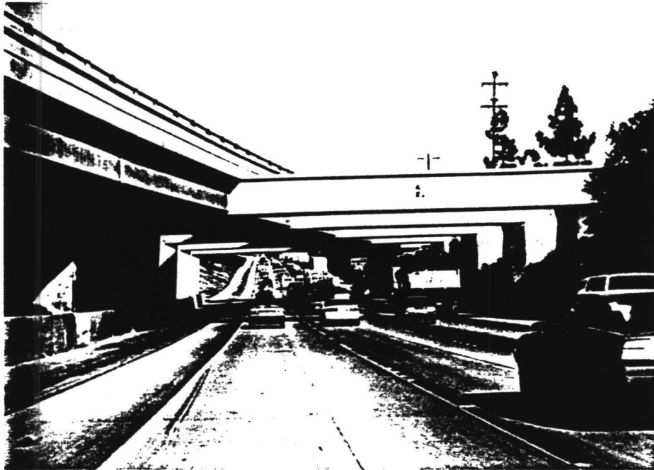
Plate 5.2 A similar use of straddle bents to transition an aerial guideway into the median of a freeway.
