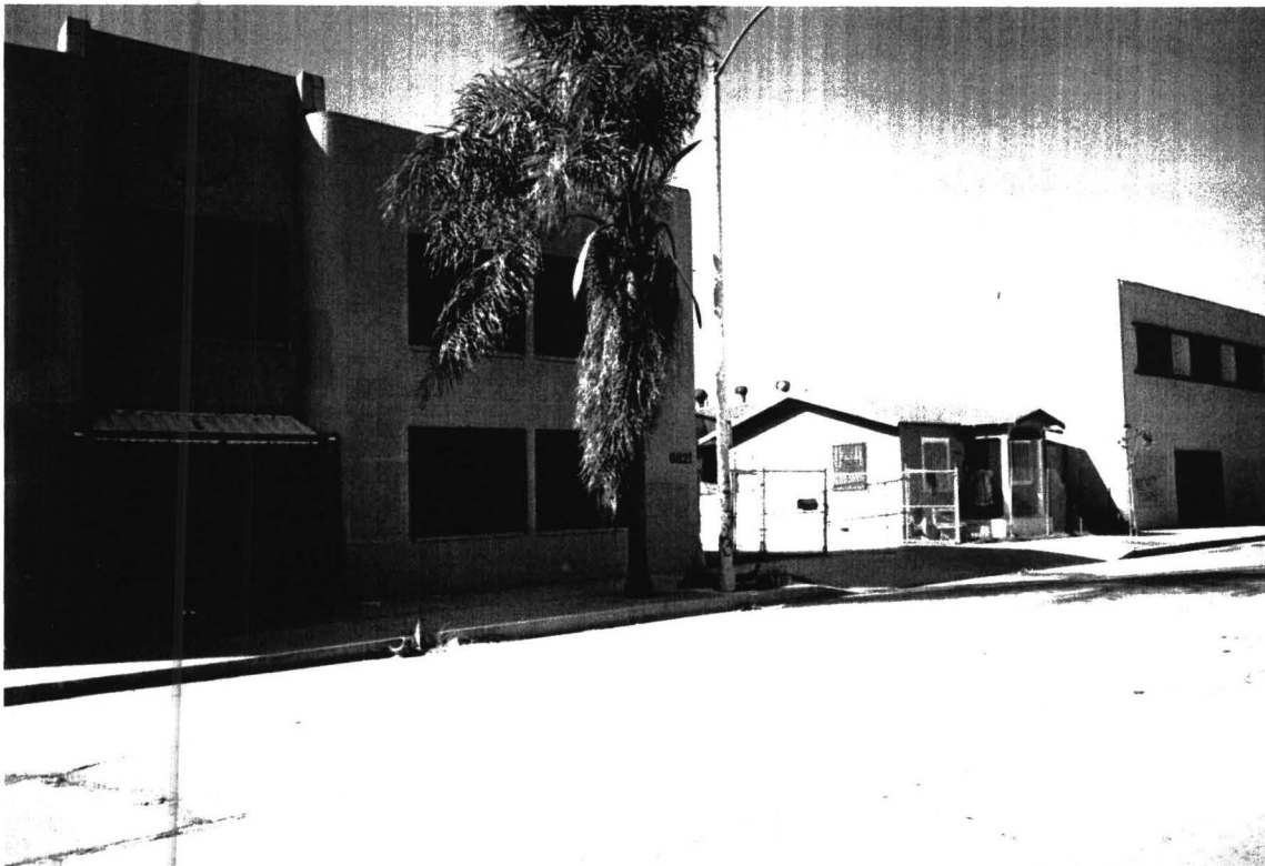
Single-family dwelling located between industrial buildings in Subarea 6 near Florence Avenue.
