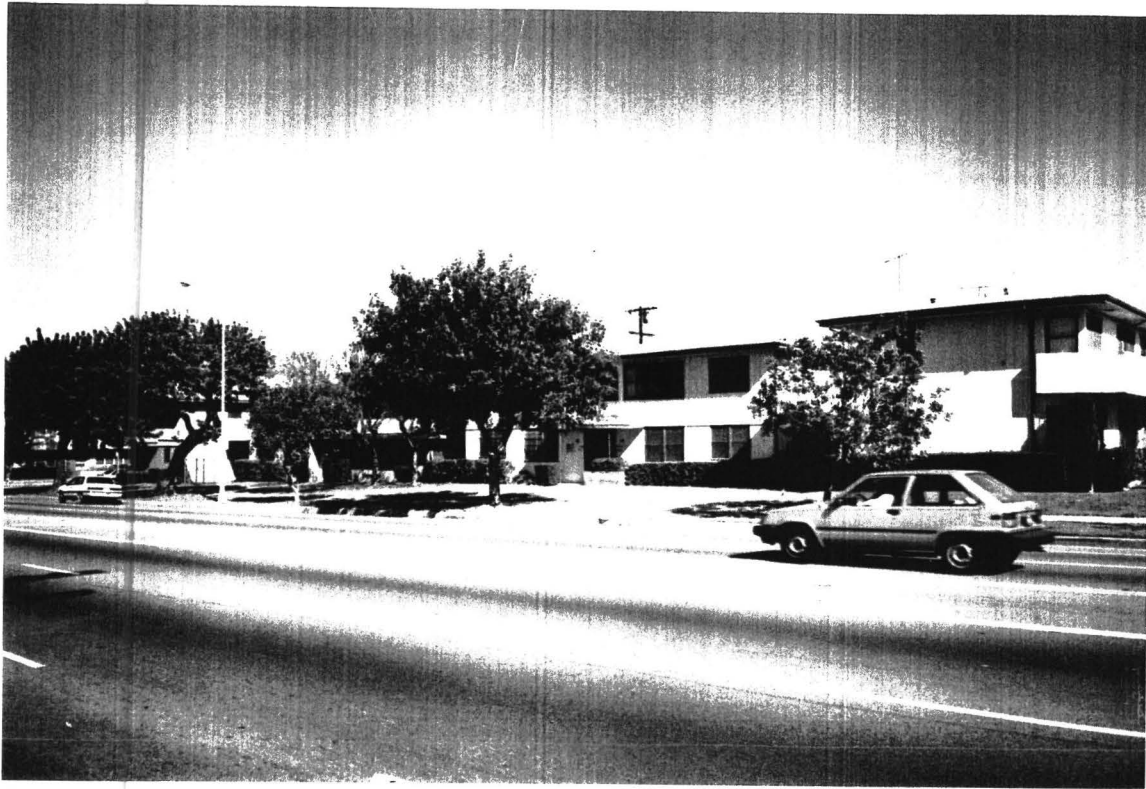
Multi-family housing located south of Florence Avenue.
