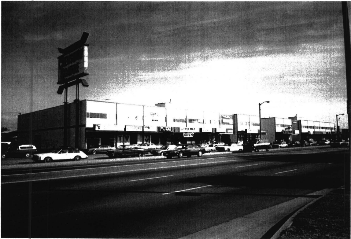
Example of office space on the second floor near 39th Street and Crenshaw Boulevard.
