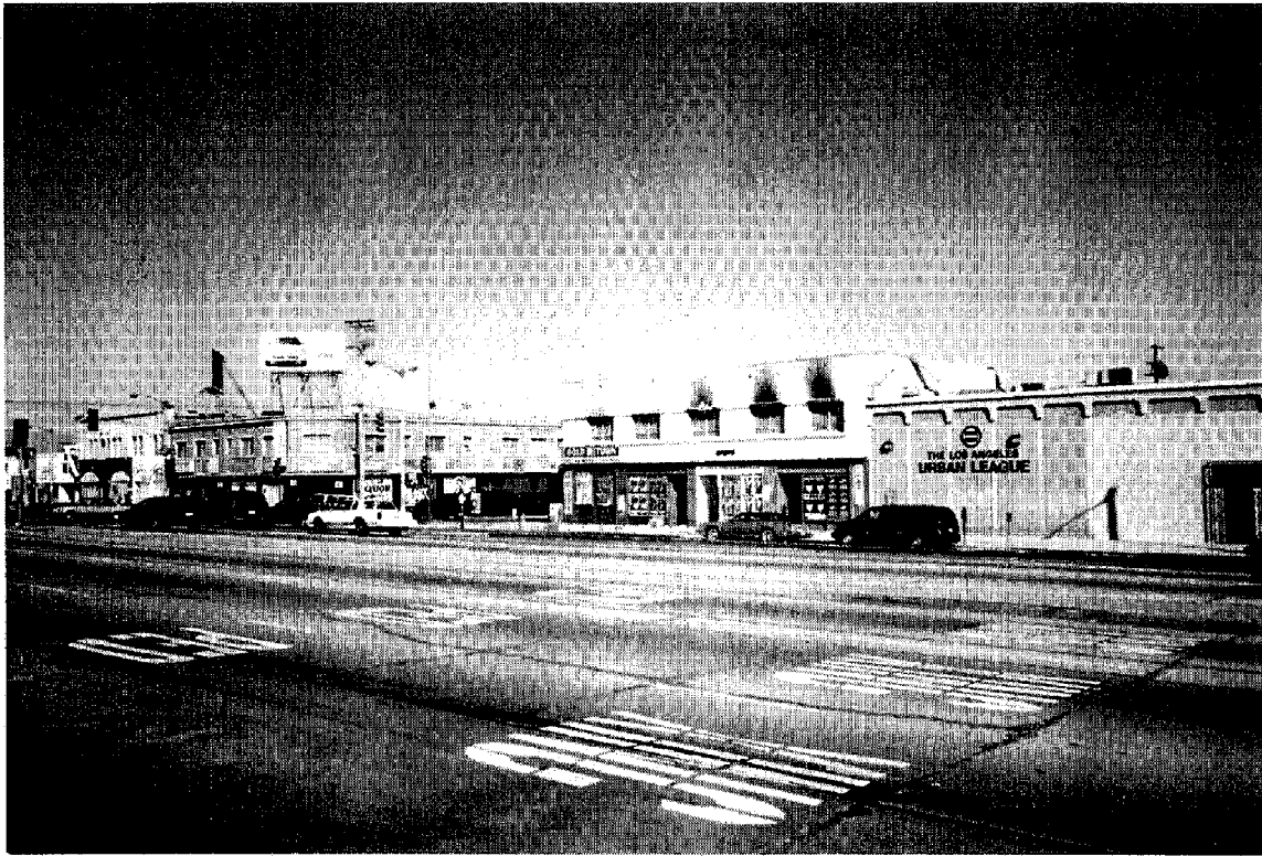
Fire damaged building at 54th Street and Crenshaw Boulevard.
