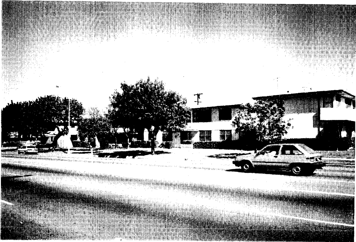
Multi-family housing located south of Florence Avenue.
