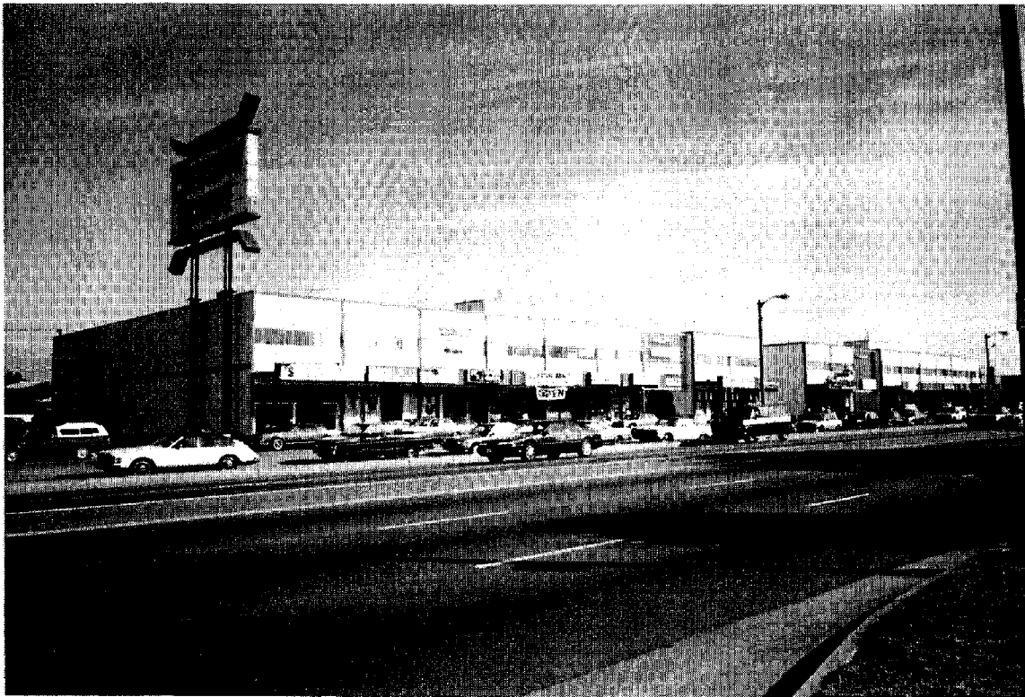
Example of office space on the second floor near 39th Street and Crenshaw Boulevard.
