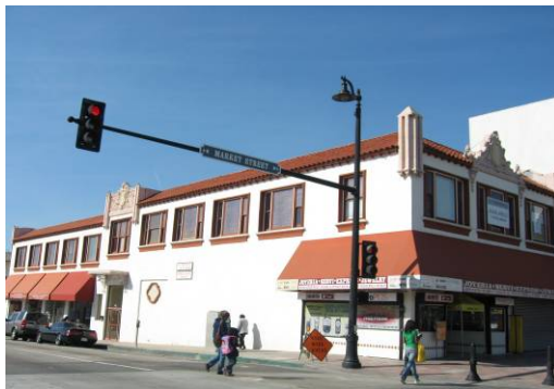
Buildings and pedestrian-oriented streetscape located in downtown Inglewood along Market Street. (E3)
