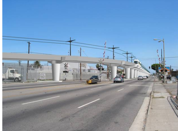
The elevated structure reduces the openness of north-south views along Crenshaw Boulevard. The elevated structure would add new visual elements. The elevated structure would be somewhat compatible with adjoining industrial land uses. (N1)
