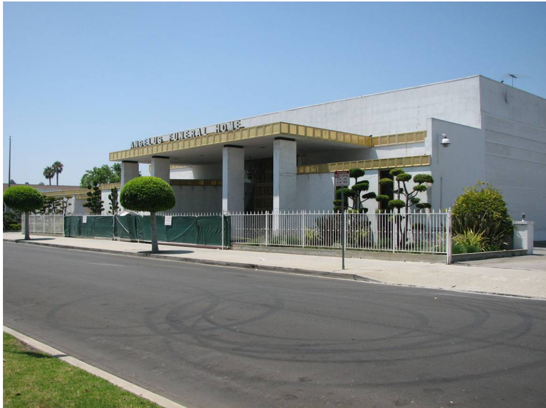
Figure 4-35. Angelus Funeral Home – 3886 Crenshaw Boulevard
