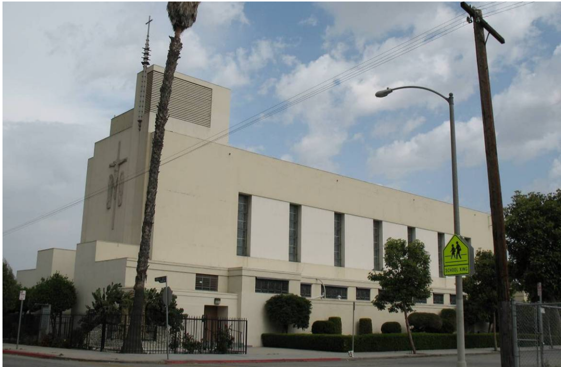
Figure 4-42. St. John the Evangelist Catholic Church – 6028 South Victoria Avenue
