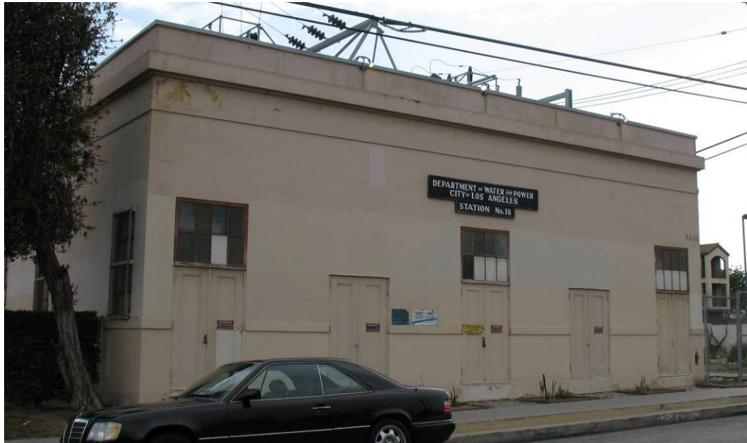
Figure 4-43. DWP Transformer Station #18 – 3316 West 60th Street
