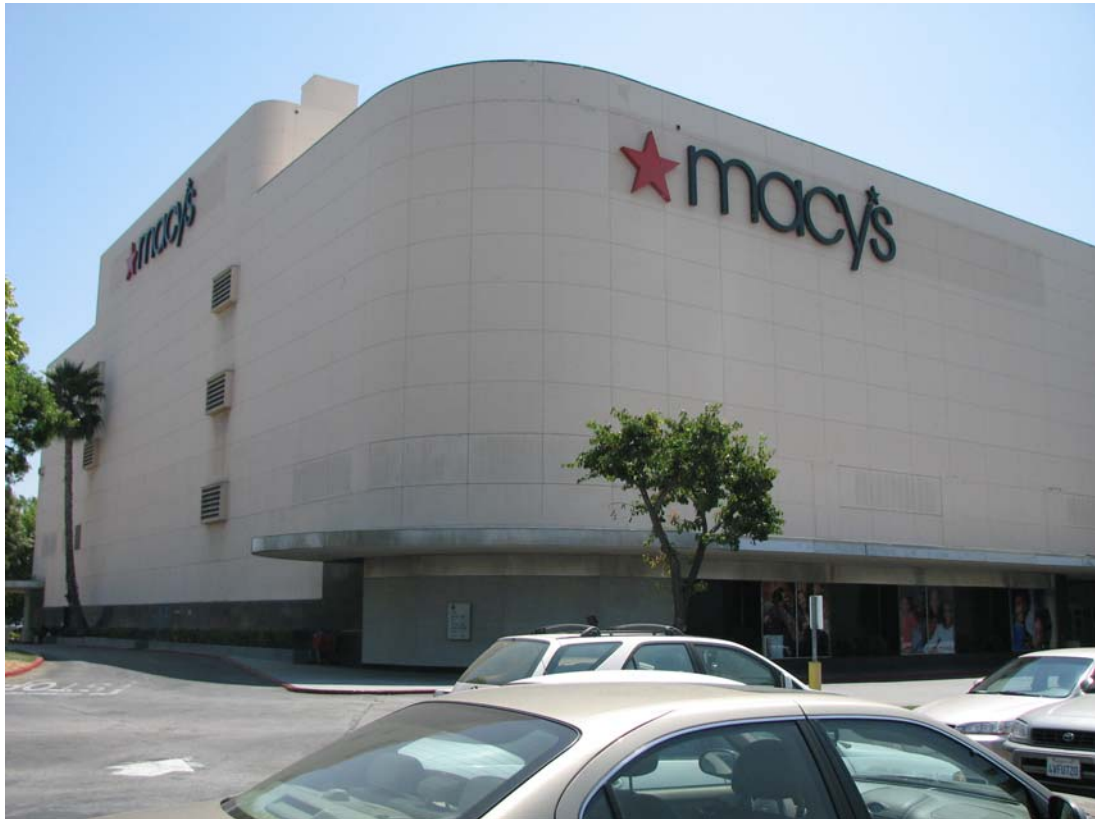
Figure 4-37. May Company Department Store (now Macy's) – 4005 Crenshaw Boulevard
