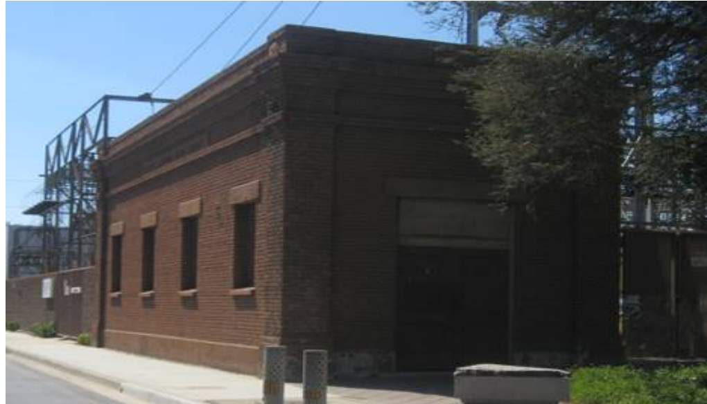
Figure 4-32. Edison Transformer House – 200 Block of West Florence Avenue
