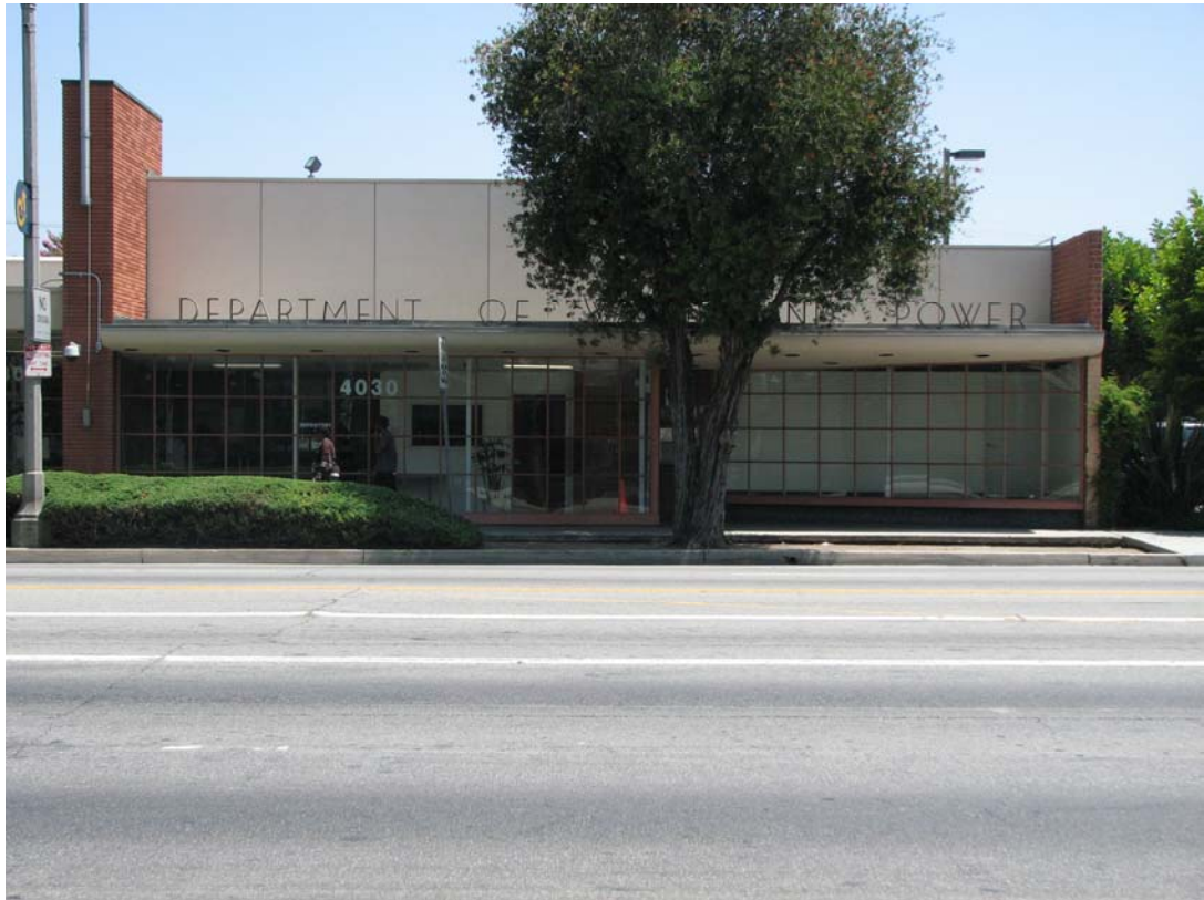
Figure 4-36. Department of Water and Power – 4030 Crenshaw Boulevard
