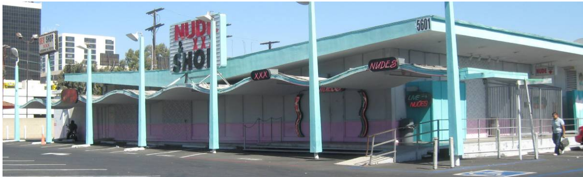
Figure 4-33. Century Lounge (formerly Carolina Lanes Bowling Center) – 5601 West Century Boulevard
