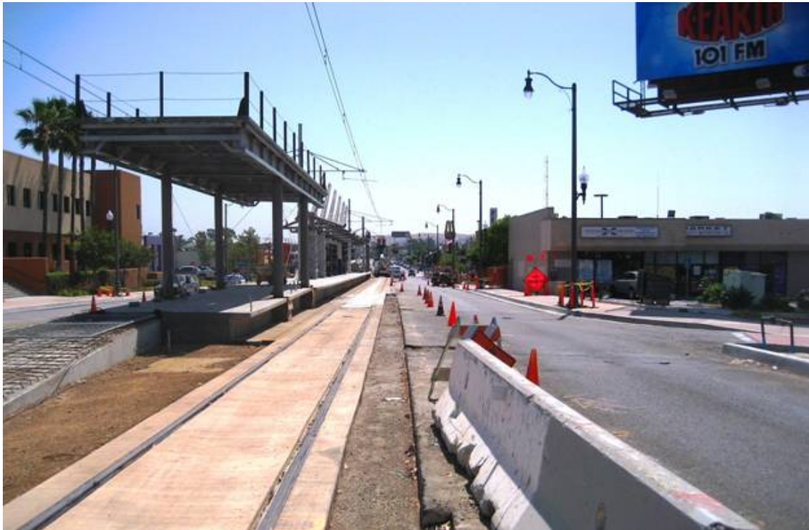
Figure 3-18. At-Grade LRT Construction
