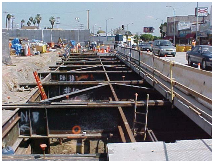
Cut and Cover Construction Gold Line Eastside Extension.
