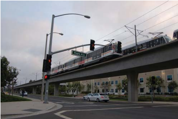
The Crenshaw LRT Alternative would travel southbound to Aviation and Imperial where it would continue south, connecting with the existing Metro Green Line, with service to the Mariposa, El Segundo, Douglas and Redondo Beach Green Line stations. Here the Metro Green Line is shown at Maple Street, just north of the Mariposa Station.
