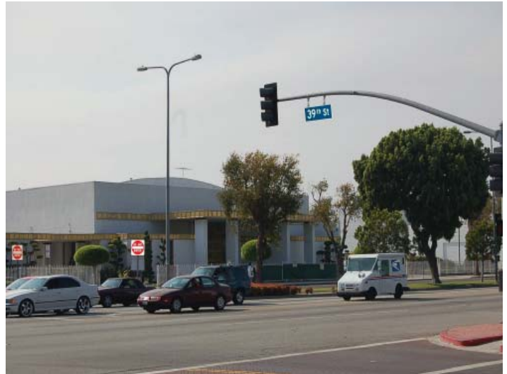
The Base LRT Alternative would have a portal to transition from surface level to below surface near 39th Street. There are a number of adjacent land uses that would be affected by this transition area.
