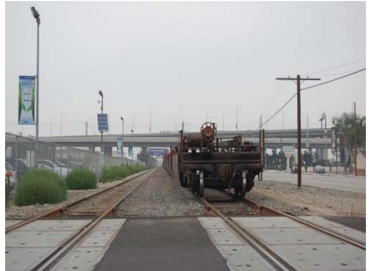
Harbor Subdivision. Continued freight use of the Harbor Subdivision poses many constraints to the development of both BRT and LRT transit service within the railroad right-of-way.
