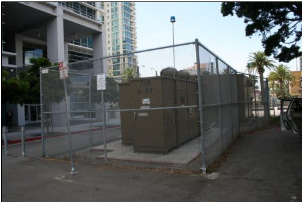
Figure 4-6: Example of a Typical TPSS
