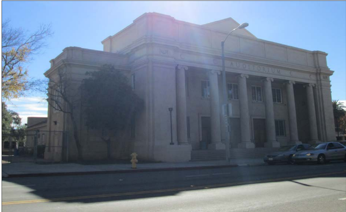
Figure 3-2: 130 N. Brand Boulevard, Auditorium, view looking southwest
