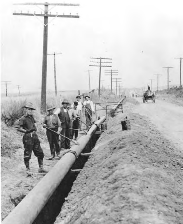
Gas line along San Fernando Road, 1910 CSUN Oviatt Library Digital Collection - San Fernando Valley History Digital Library
