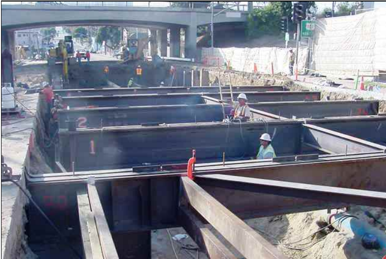
Figure 2-10: Example of Tunnel Portal Beam Installation
