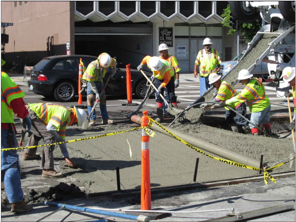
Figure 2-2: Concrete Pour for Bus Lane Surface
