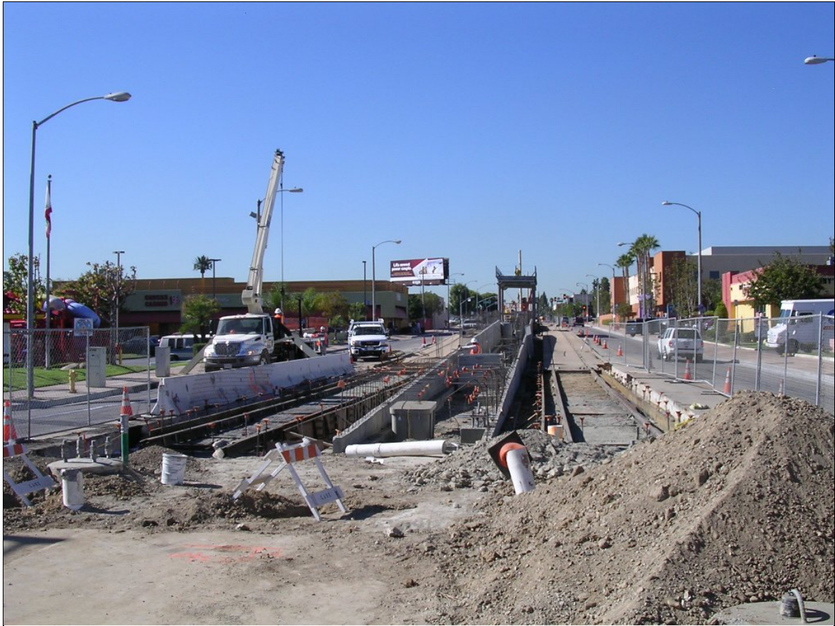
Figure 2-8: Example of Street Median LRT Station Construction
