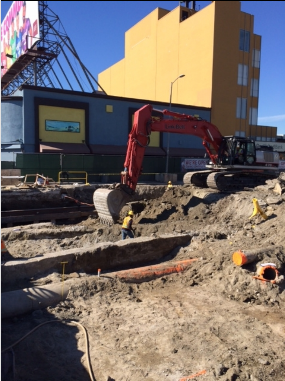
Figure 2-9: Example of In-Street Excavation
