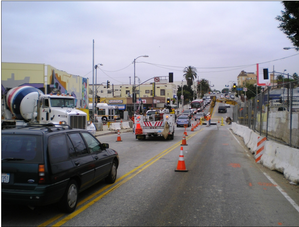
Figure 2-4: Example of Temporary Traffic Control at Intersections During Construction
