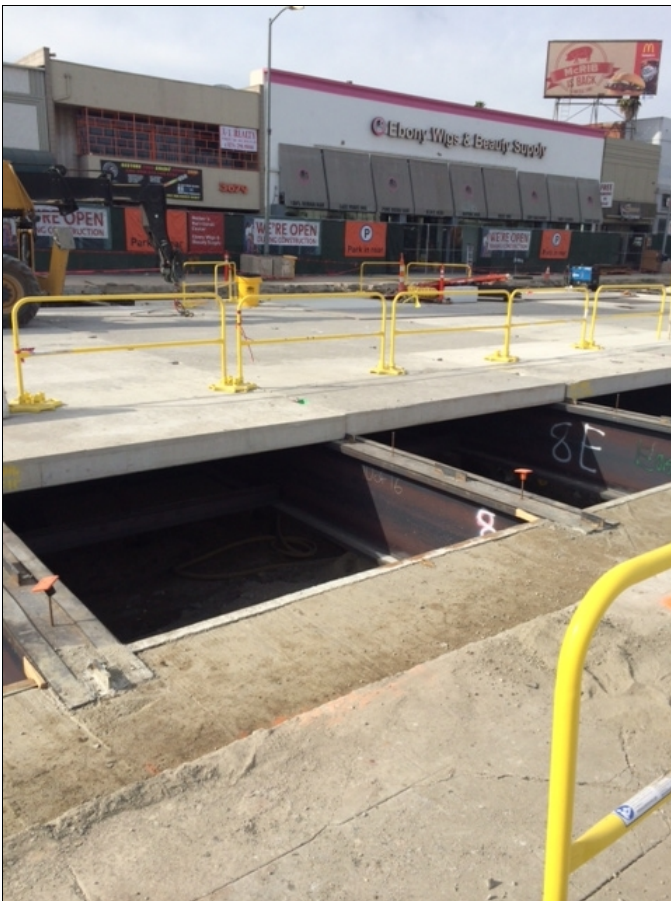
Figure 2-11: Example of Tunnel Portal Decking
