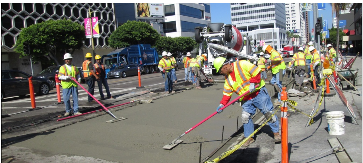
Figure 2-3: Concrete Finishing for Bus Lane Surface
