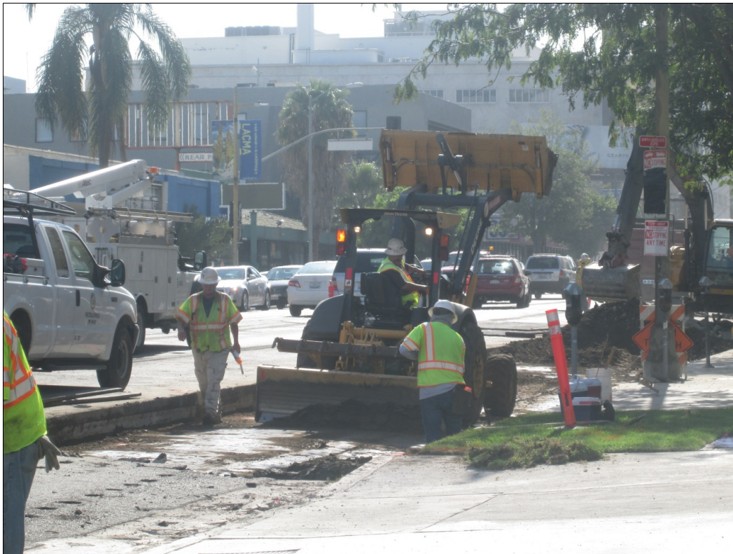
Figure 2-1: Roadway Bed Grading and Paving
