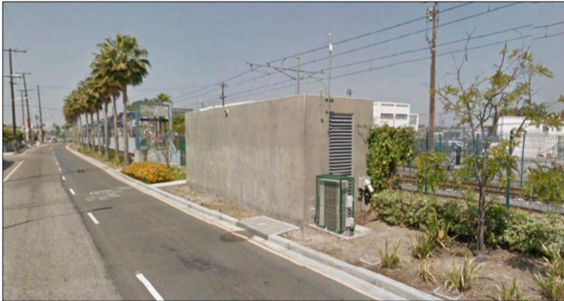
Figure 2-14: Typical TPSS for Tram/LRT
