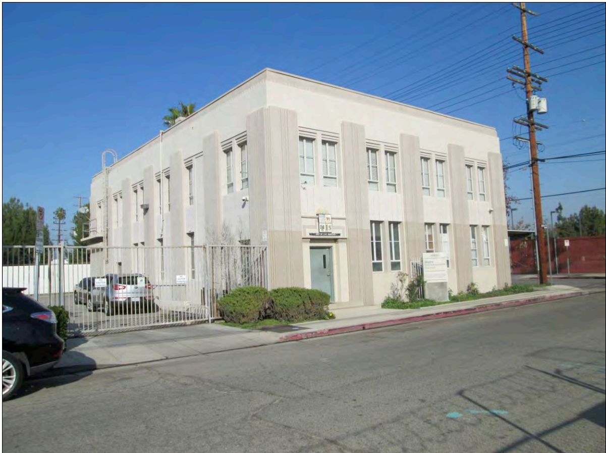
Figure 4.16-1: 14601–3 Aetna Street, view looking northeast
