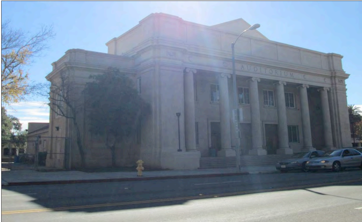
Figure 4.16-2: 130 N. Brand Boulevard, Auditorium, view looking southwest
