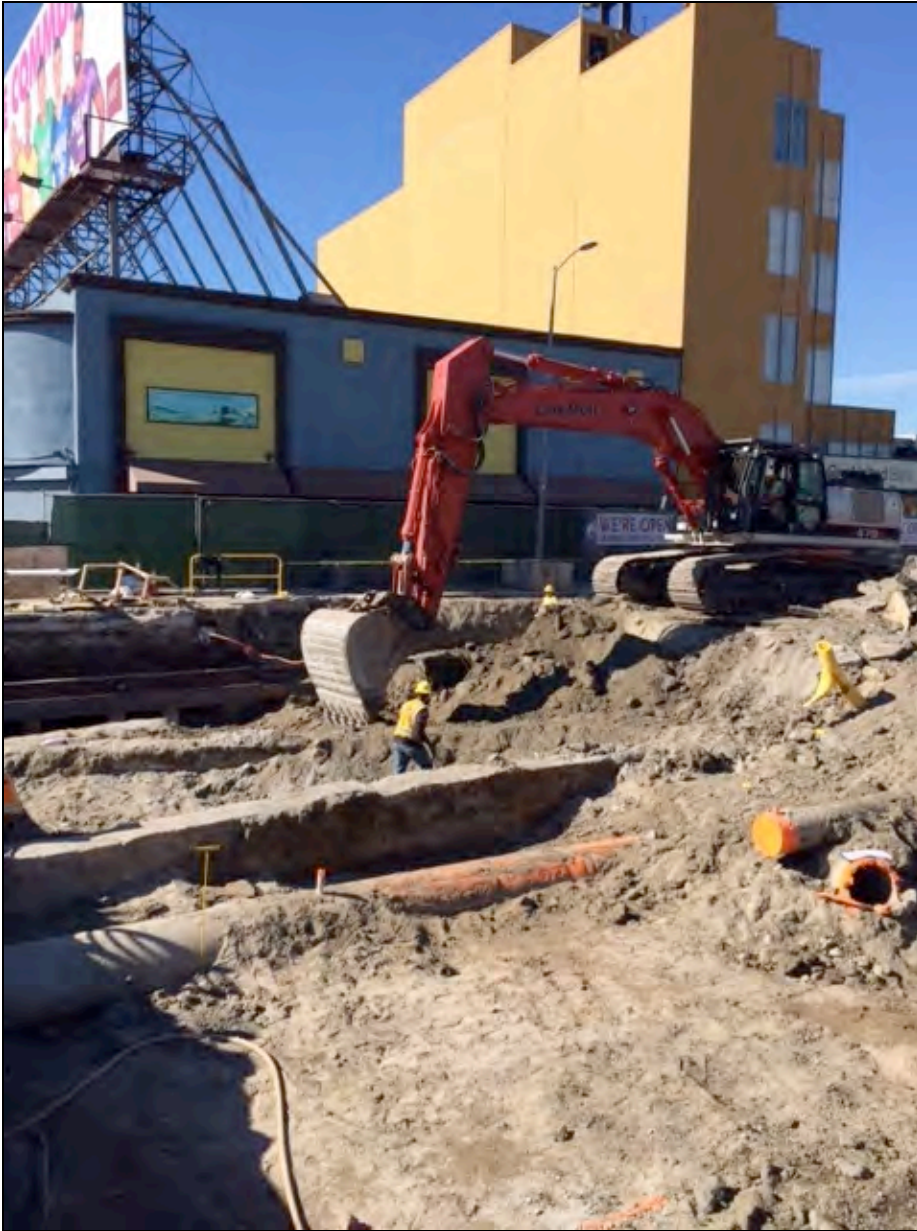
Figure 4.19-9: Example of In-Street Excavation
