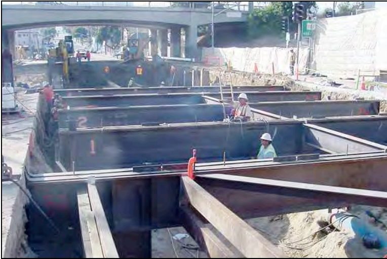
Figure 4.19-10: Example of Tunnel Portal Beam Installation
