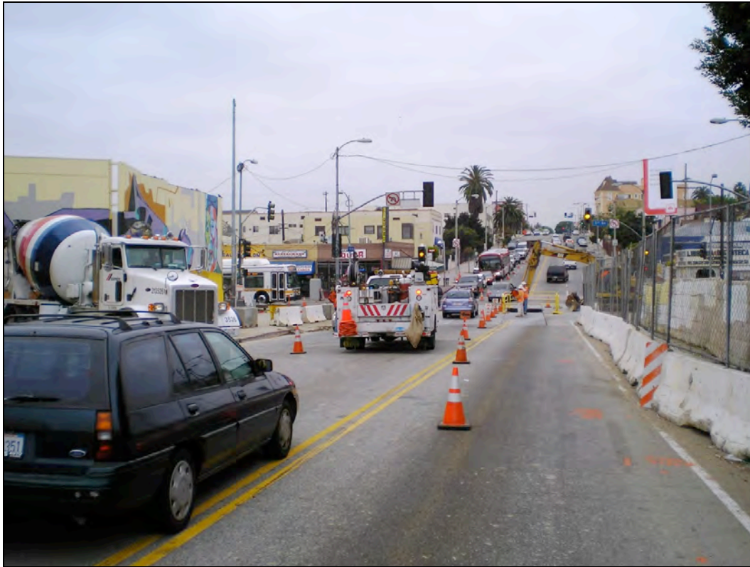
Figure 4.19-4: Example of Temporary Traffic Control at Intersections During Construction
