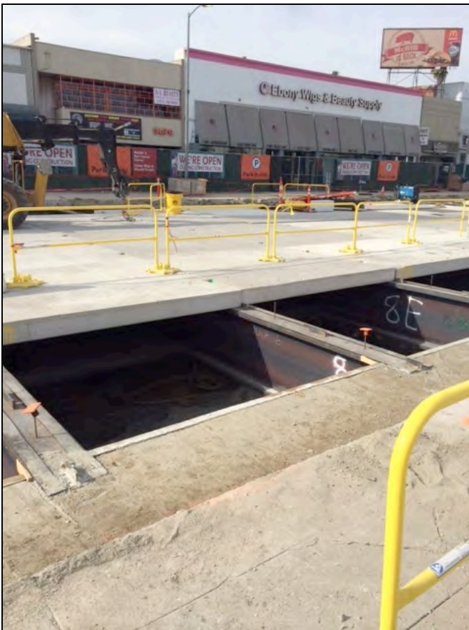
Figure 4.19-11: Example of Tunnel Portal Decking
