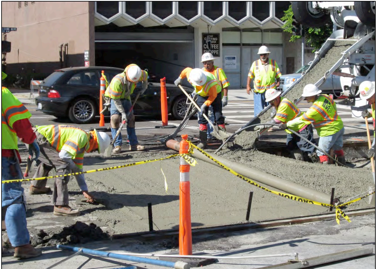
Figure 4.19-2: Concrete Pour for Bus Lane Surface
