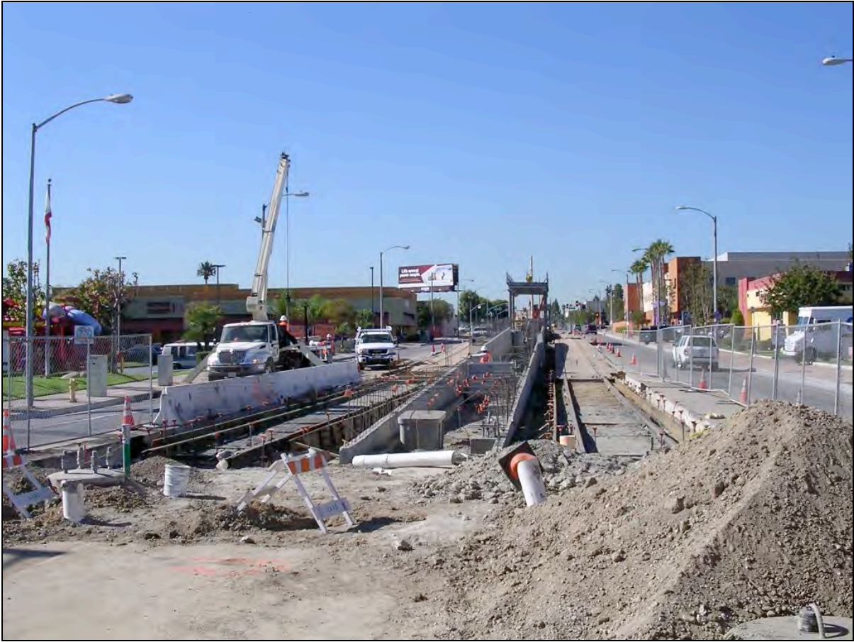
Figure 4.19-8: Example of Street Median LRT Station Construction
