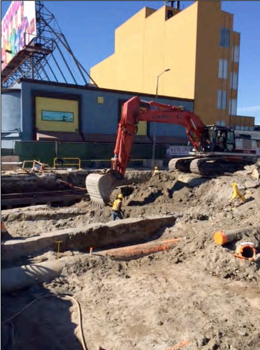
Figure 4.19-9: Example of In-Street Excavation
