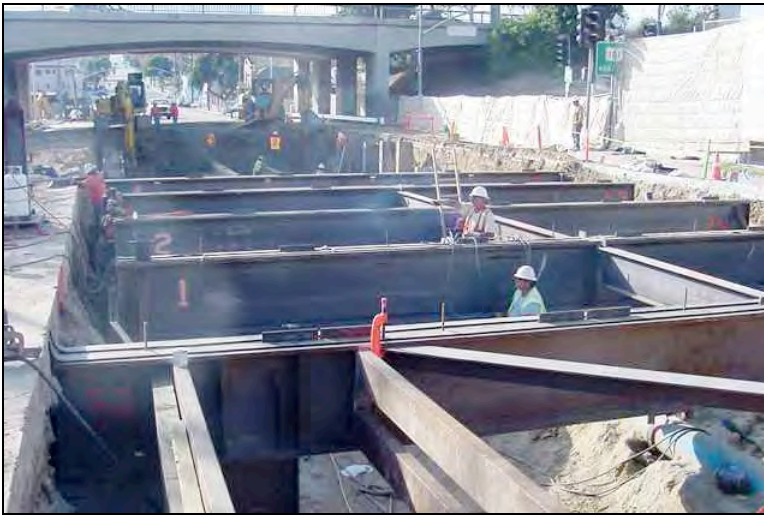
Figure 4.19-10: Example of Tunnel Portal Beam Installation
