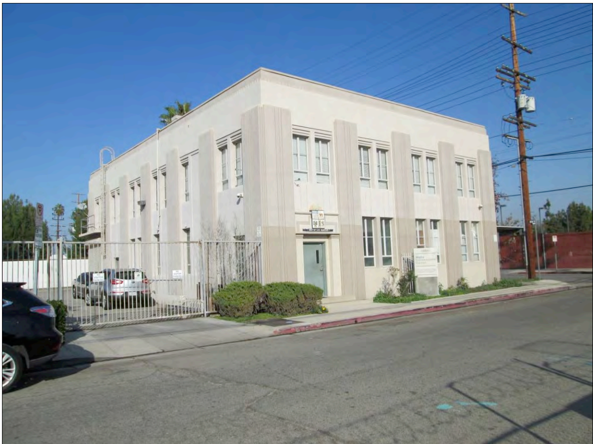
Figure 4.16-1: 14601–3 Aetna Street, view looking northeast
