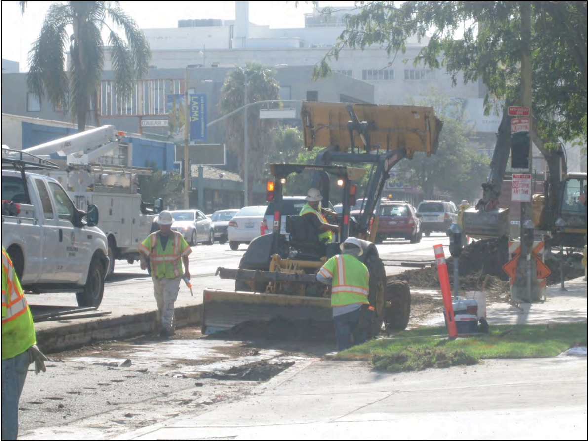
Figure 4.19-1: Roadway Bed Grading and Paving
