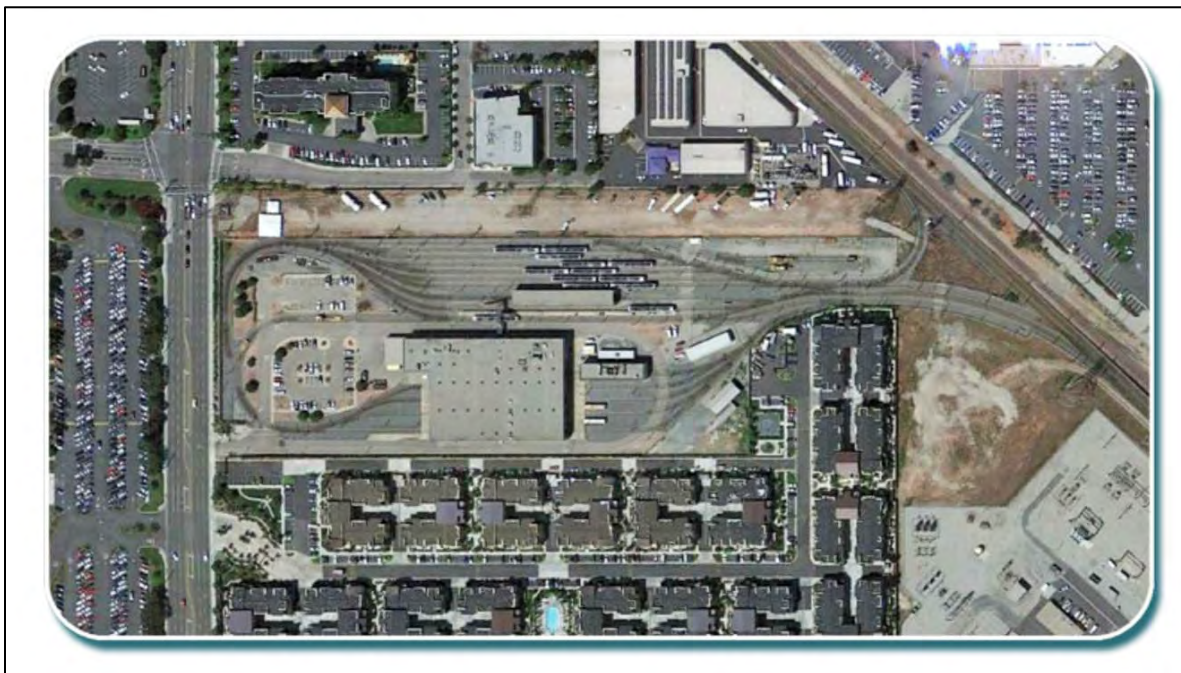
Figure 1-6: Typical MSF Site
