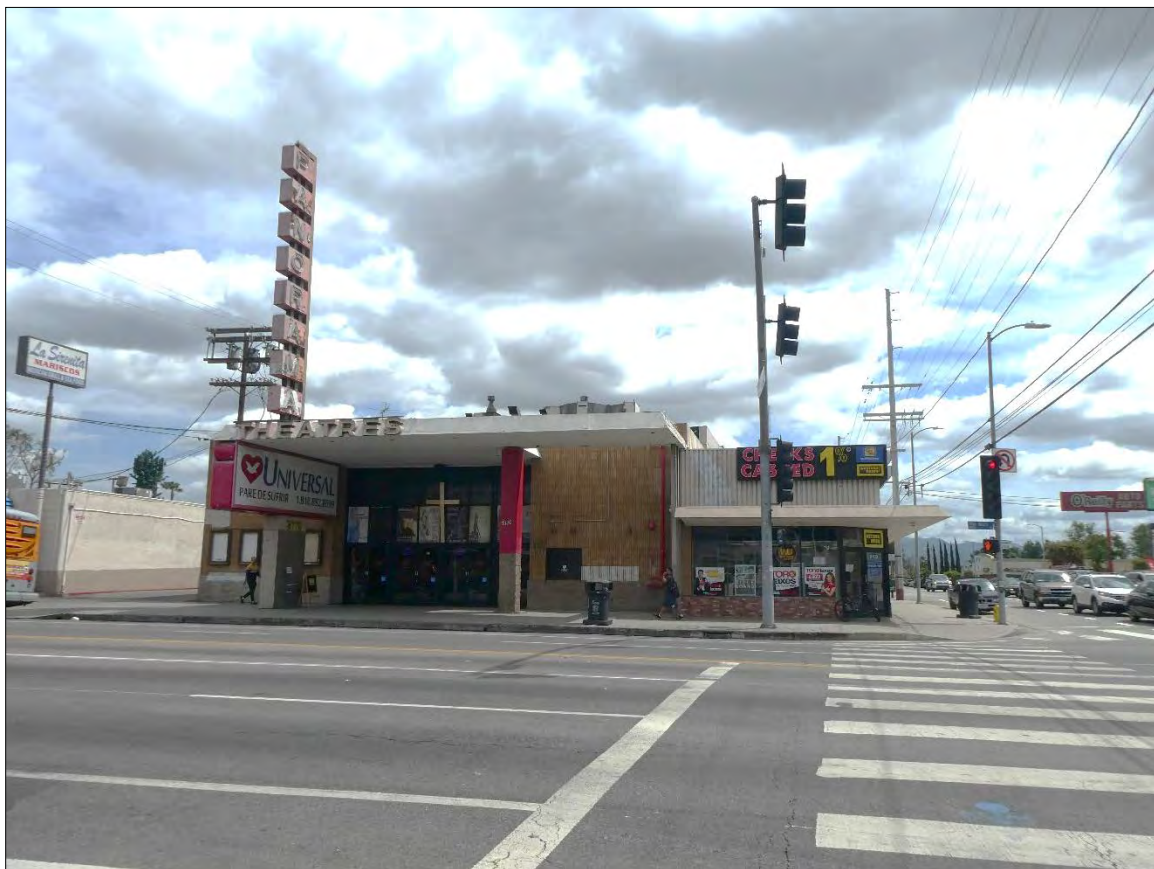
Figure 5-5: 9110 Van Nuys Boulevard, view looking east
