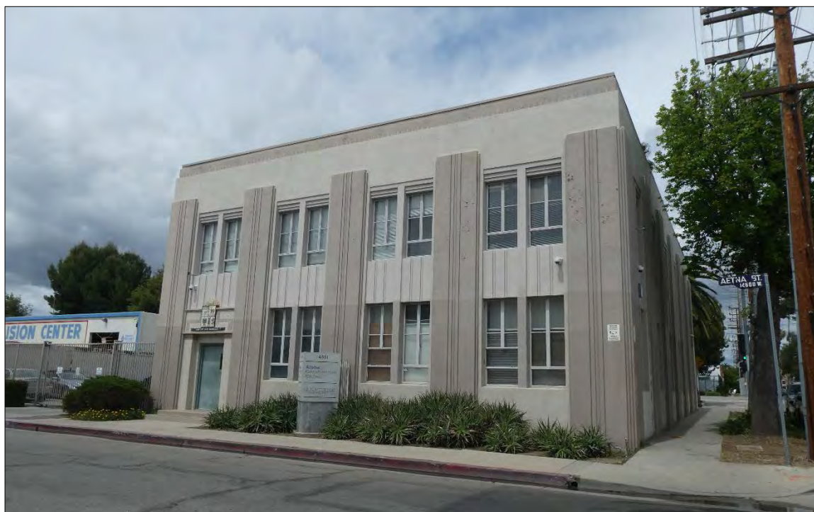
Figure 5-16: 14601 Aetna Street, view looking north
