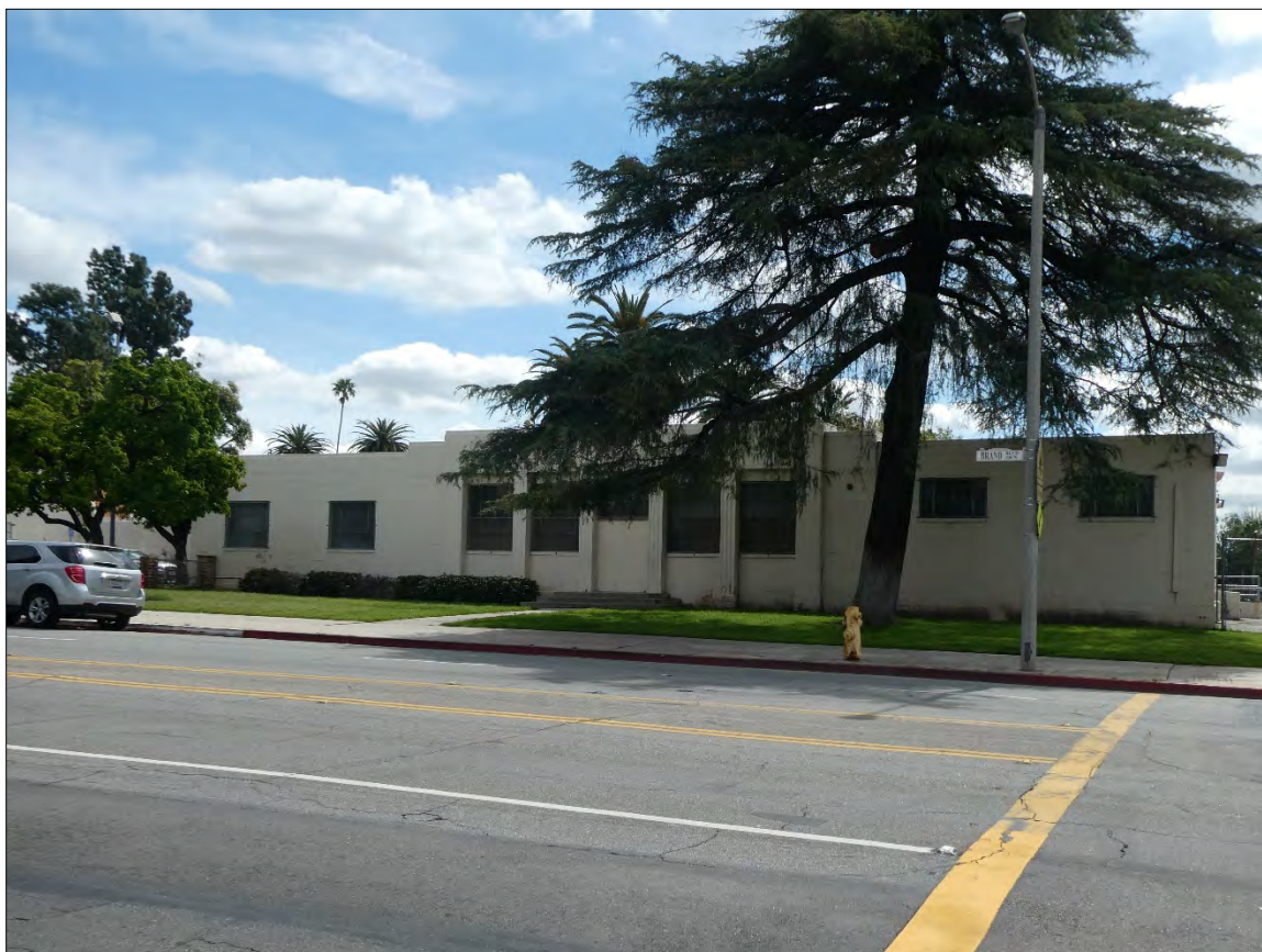
Figure 5-1: 130 Brand Avenue - Boy's Gymnasium
