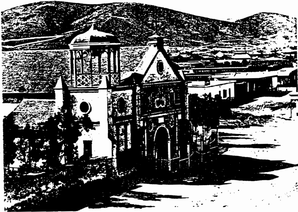
14. The pueblo church, Nuestra Señora la Reina de Los Angeles, east of the plaza in 1875. Notice how the church's architecture has been changed by Anglo-American influence. Courtesy of the Huntington Library.
