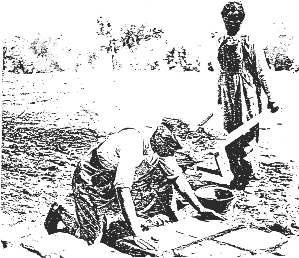
4. Adobe brick-making. Most of the Sonora Town homes built in the nineteenth century continued to be made in the traditional manner. Courtesy of the California Historical Society, Los Angeles.
