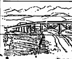
First street viaduct.
