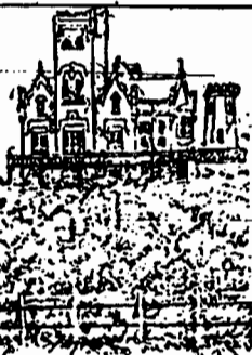
General Perry-Davis residence.
