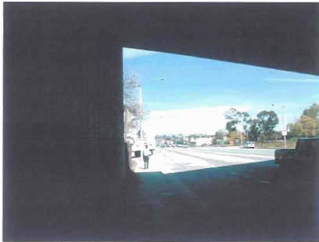
Underpass at Atlantic Boulevard under State Route 60 Freeway
