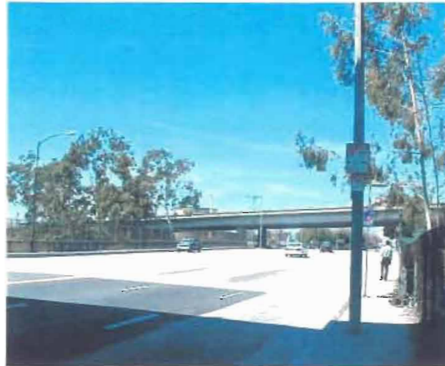
Narrow sidewalk along Ford Boulevard Bridge over 710 Freeway
