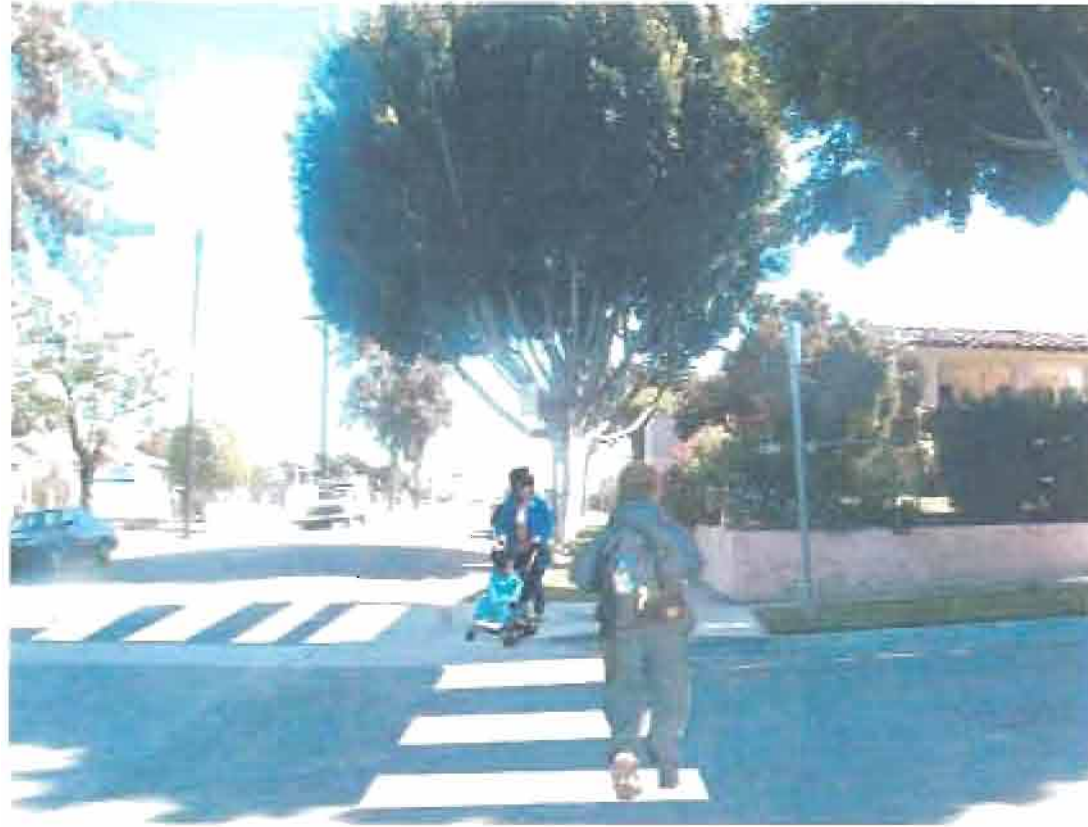
Potential typical crosswalk improvement where bulb-outs are not necessary near the Maravilla Station neighborhood
