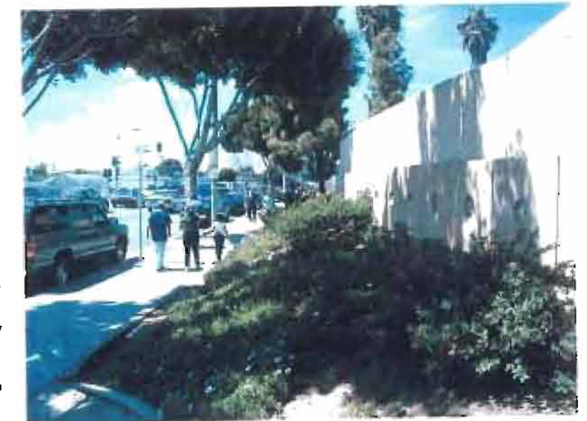
Existing narrow sidewalk on 3rd Street at Roybal Health Center
