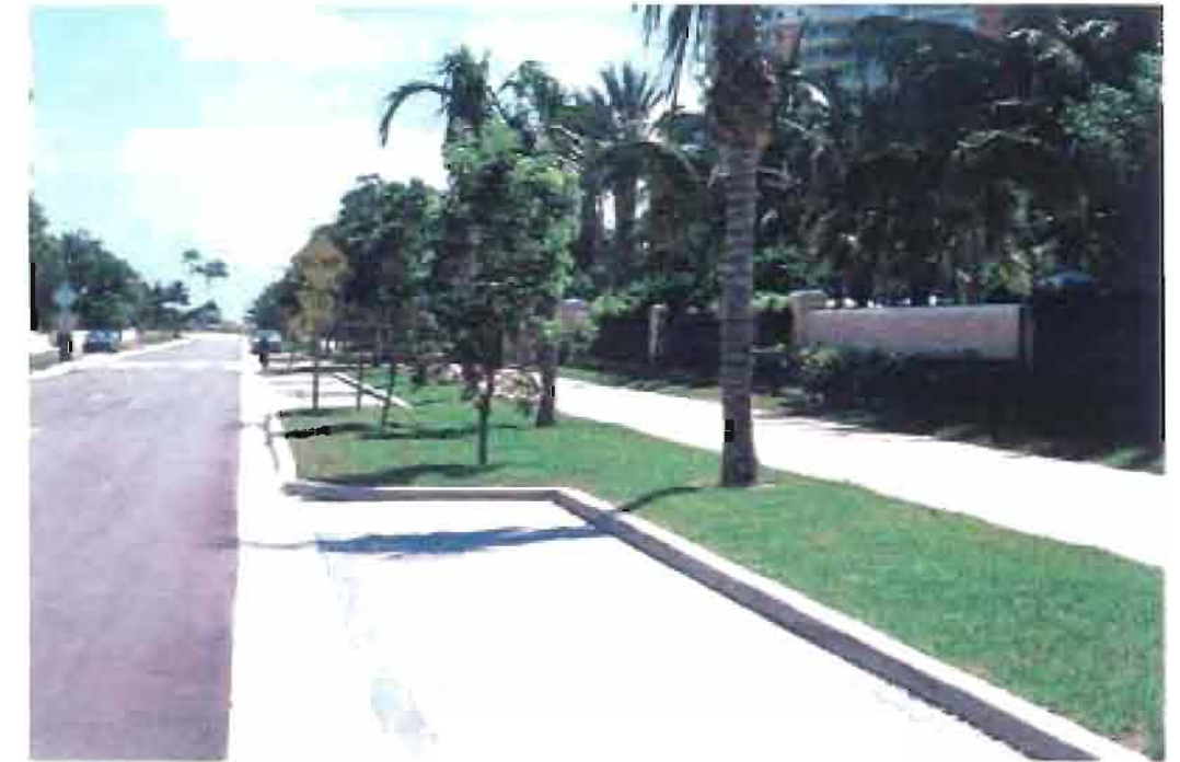
An example of a bulb-out with a valley gutter distinguishing the travel lane and parking area.
