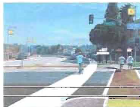
Mednik Avenue offers potential as a key connector in the County's Regional Bikeway system.
