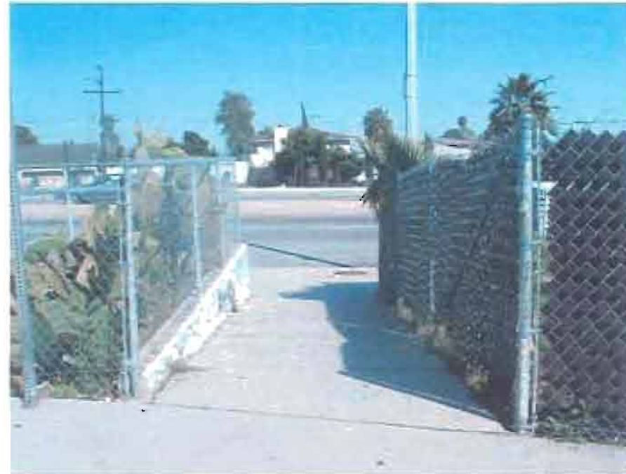
Existing pedestrian access at Strang Street and Arizona Avenue in poor condition
