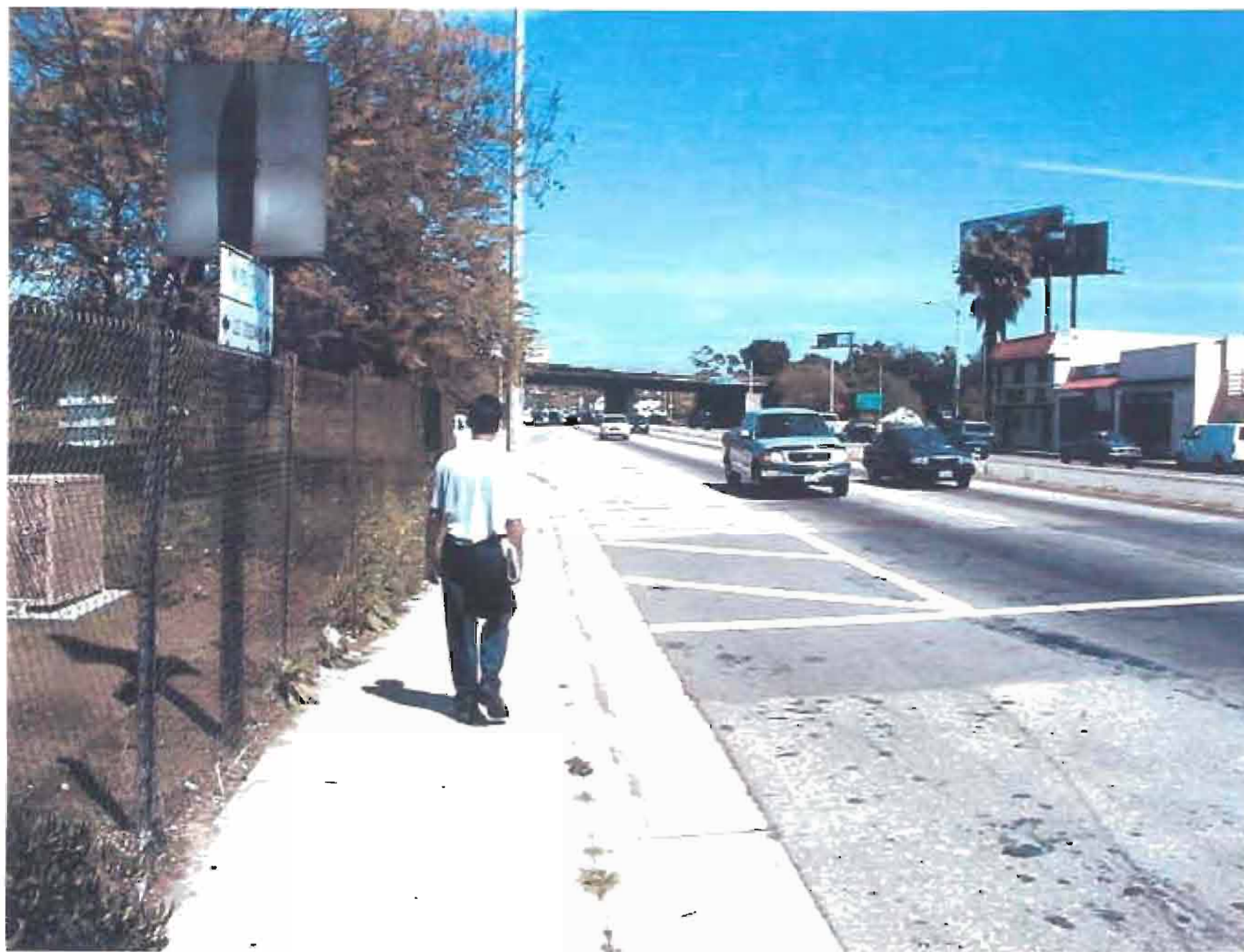
Narrow sidewalk on Atlantic Boulevard
