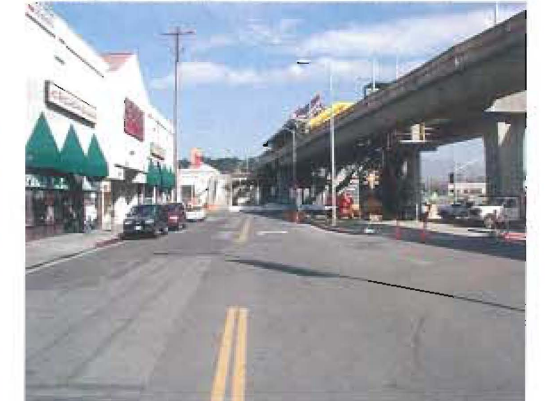
04. Alameda Street looking towards Chinatown Station
