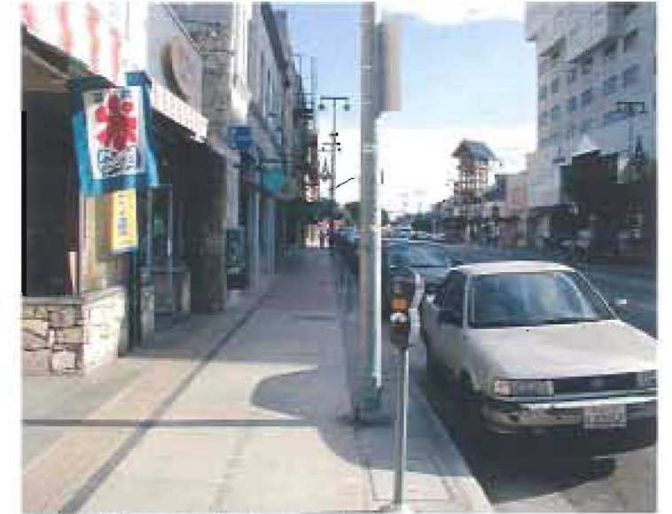
04. First Street north sidewalk paving
