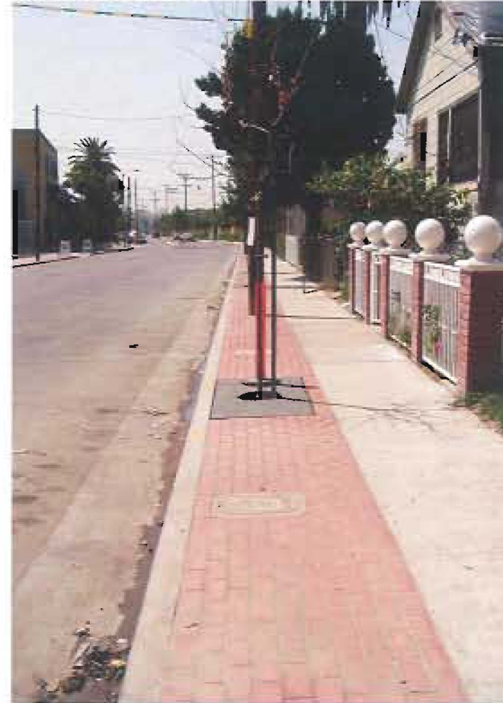
06. Pico Alto Pedestrian Linkages sidewalk paving
