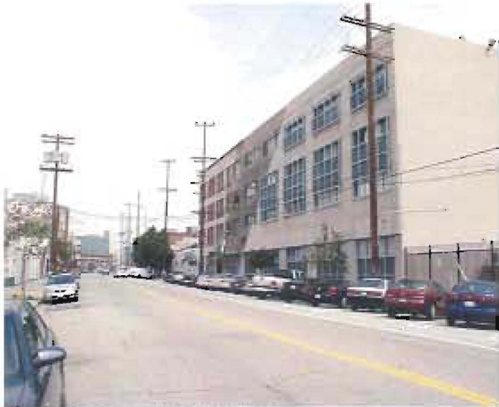
01. Traction Avenue looking west
