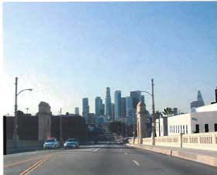
01. First Street bridge looking towards downtown
