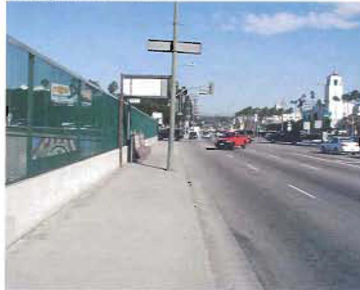
05. Bridge over 10 freeway
