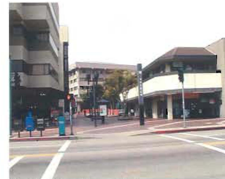
03. Second Street JAGCC entrance
