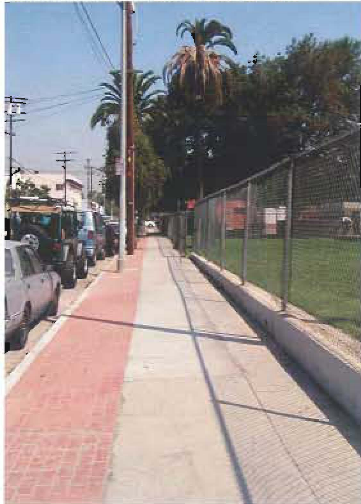
05. Pico Alto Pedestrian Linkages sidewalk paving
