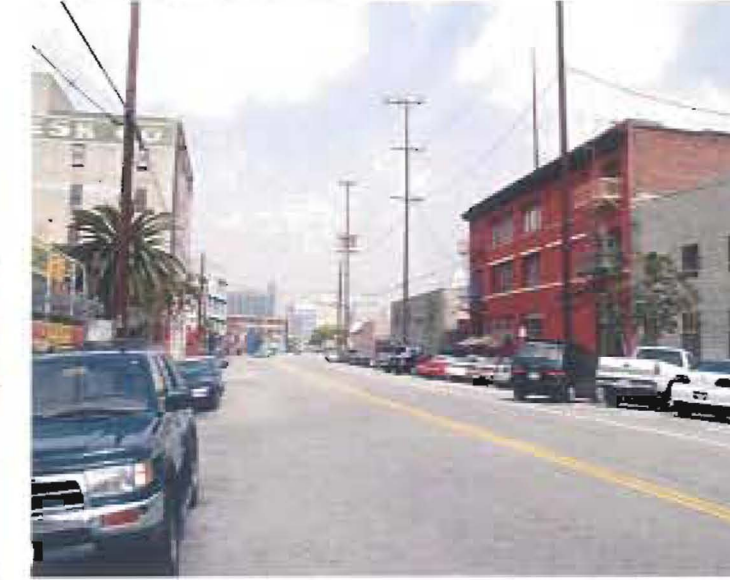
06. Traction Avenue looking west
