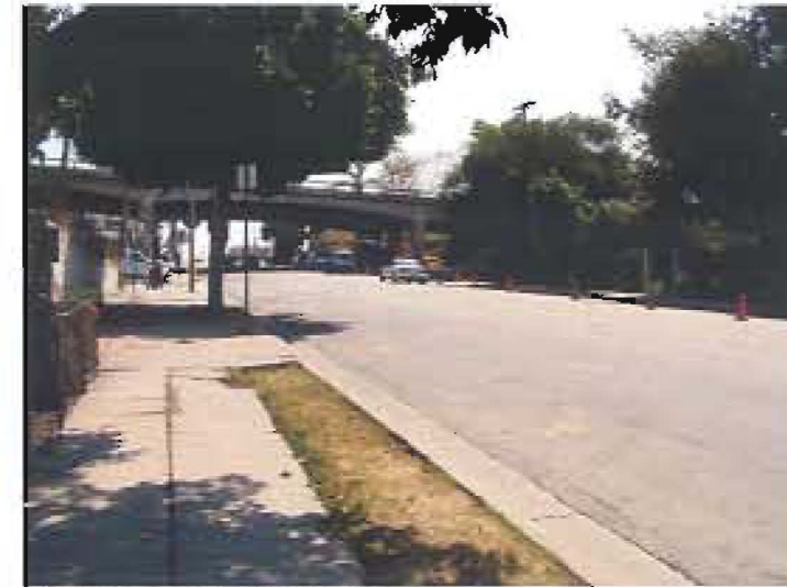
03. First Street West Portal location
