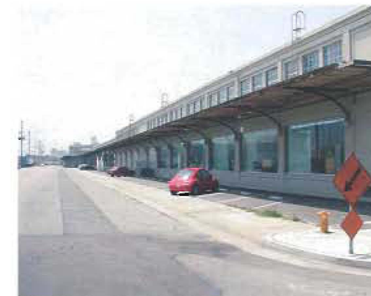
02. Traction Avenue SCI-ARC Building
