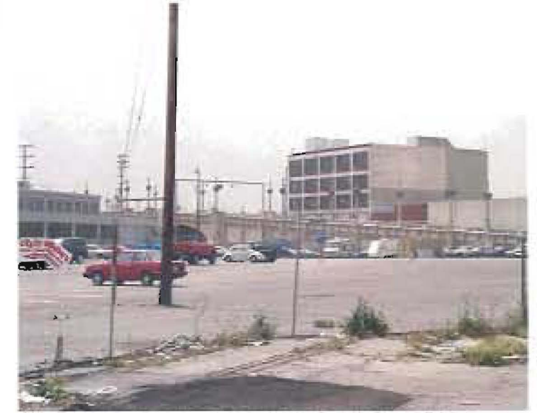
04. End of Traction looking towards Fourth Street Bridge
