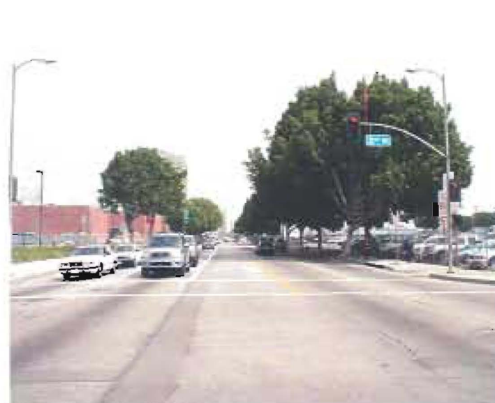
02. Alameda looking north
