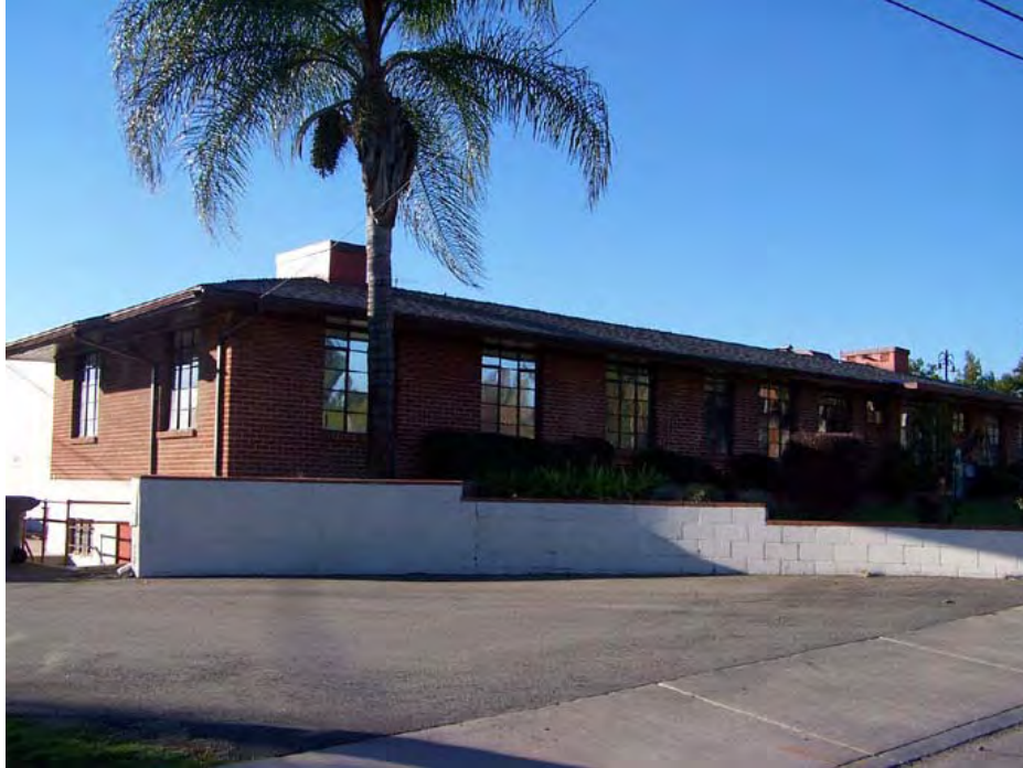
111 S. College Avenue. Facing the southeast facades. The storefront type building constructed in 1960.
