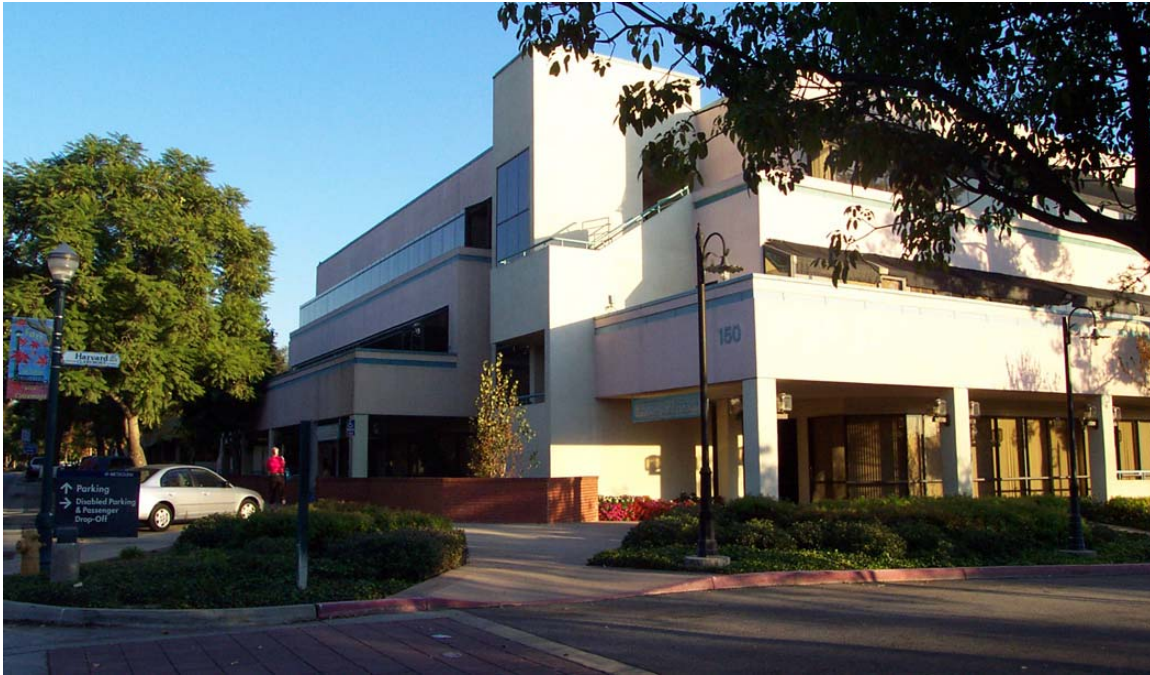
Figure 3-17.21: Claremont, Office Development Adjoining Railroad Station, View E
