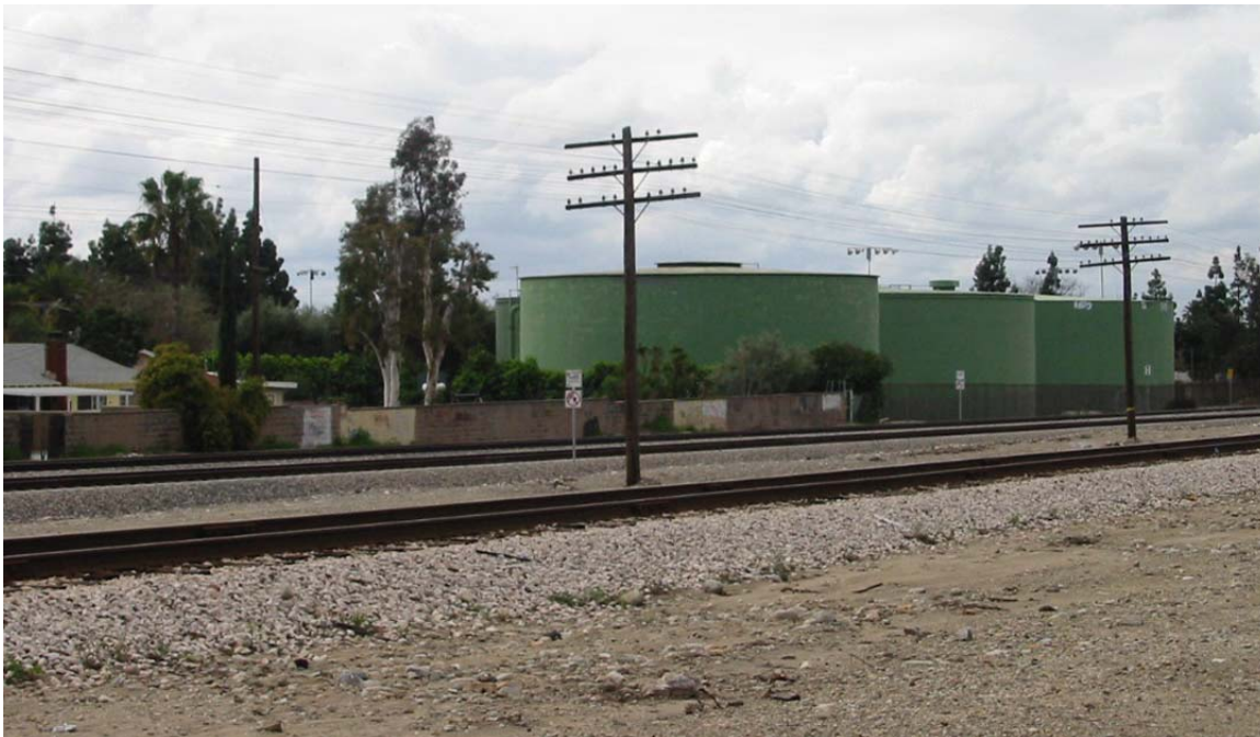
Figure 3-17.20: Pomona, Railroad Right-of-Way, Rear of Park, View SW
