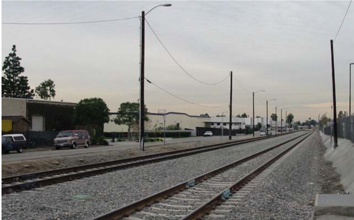
Figure 3-17.18: Pomona, Railroad Right-of-Way, View W to Metrolink Station
