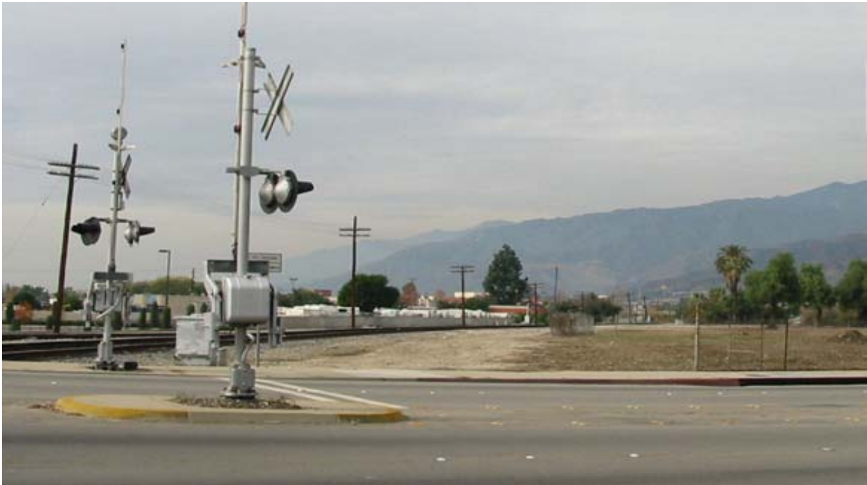
Figure 3-17.11: Glendora, Setting of Proposed Station, View W from Glendora Ave.
