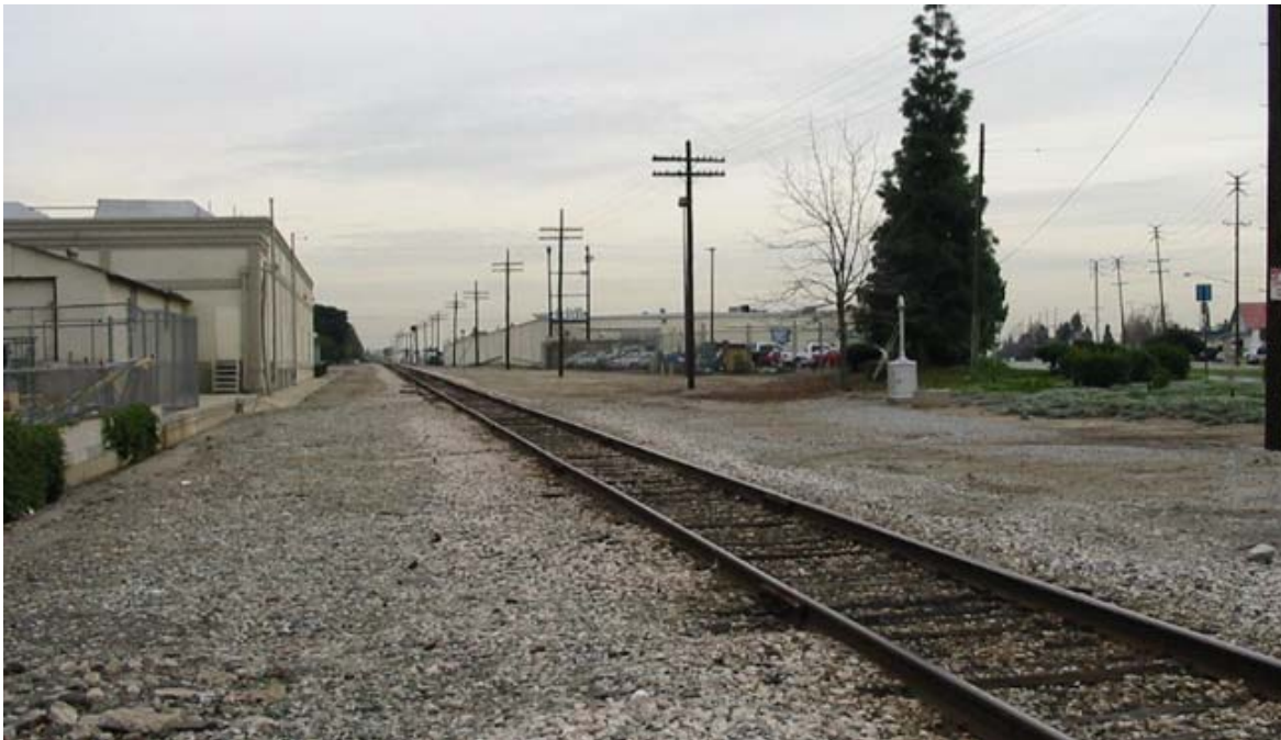
Figure 3-17.17: La Verne, View E along Railroad Right-of-Way from E Street
