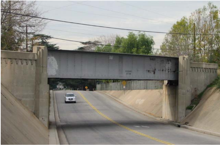
Figure 3-17.1: Arcadia, Railroad Crossing, at W. Colorado Blvd.
