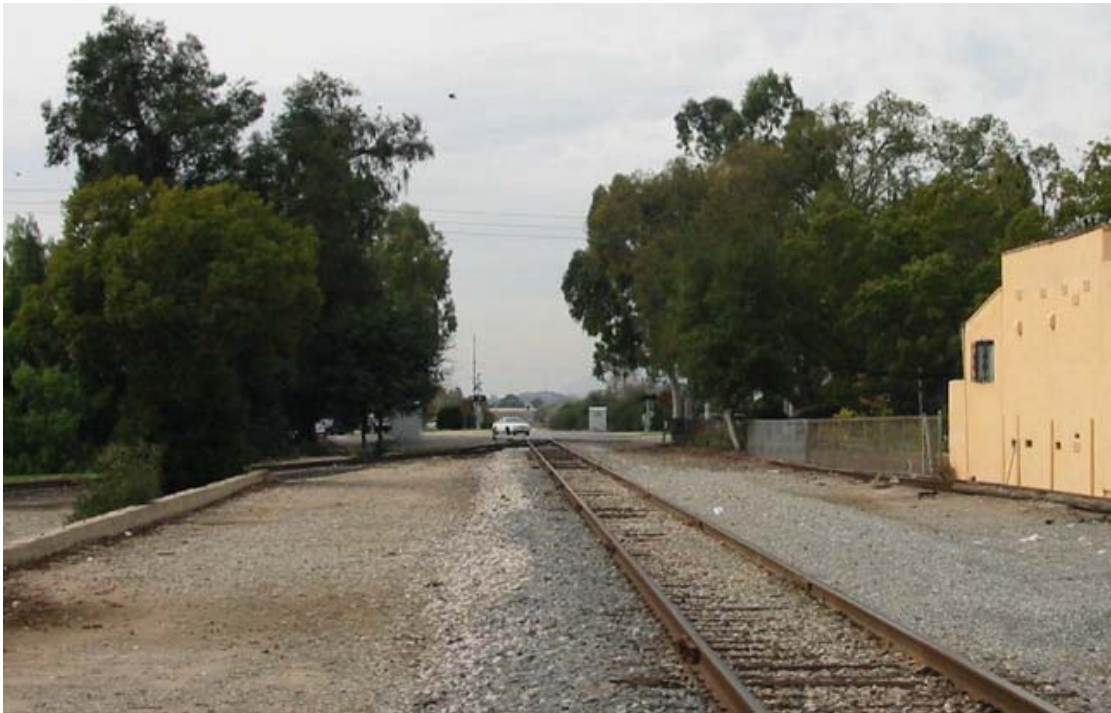
Figure 3-17.14: San Dimas, View NW from ATSF Depot to LRT Station Site
