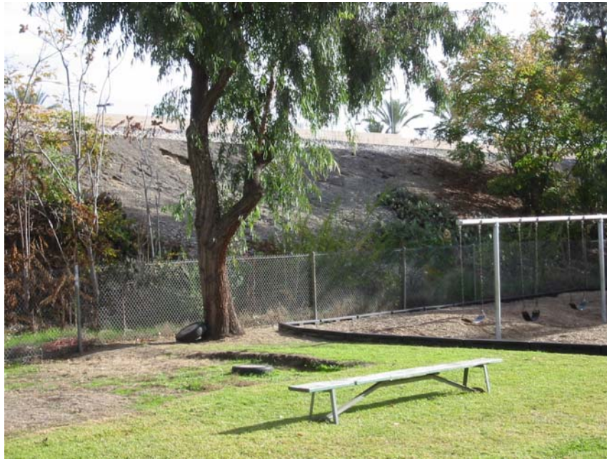
Figure 3-4.5: View of Serendipity School Playground Fence, Railroad Right-of-Way, and Raised Berm
