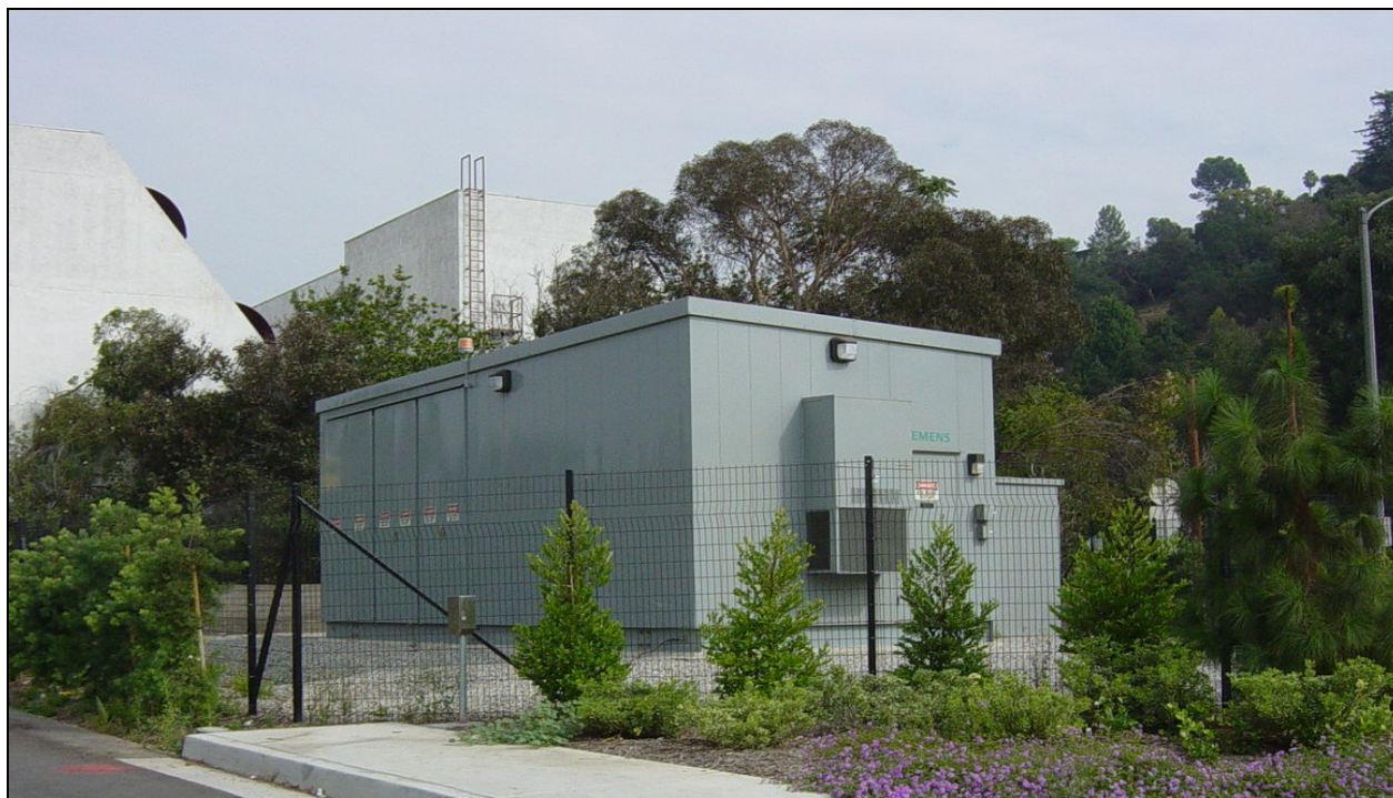
Figure 2-50: Typical Existing TPSS Facility Located on Gold Line Phase I
