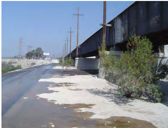
Figure 4.1-9: San Gabriel River Bridge Replacement Site View 9
