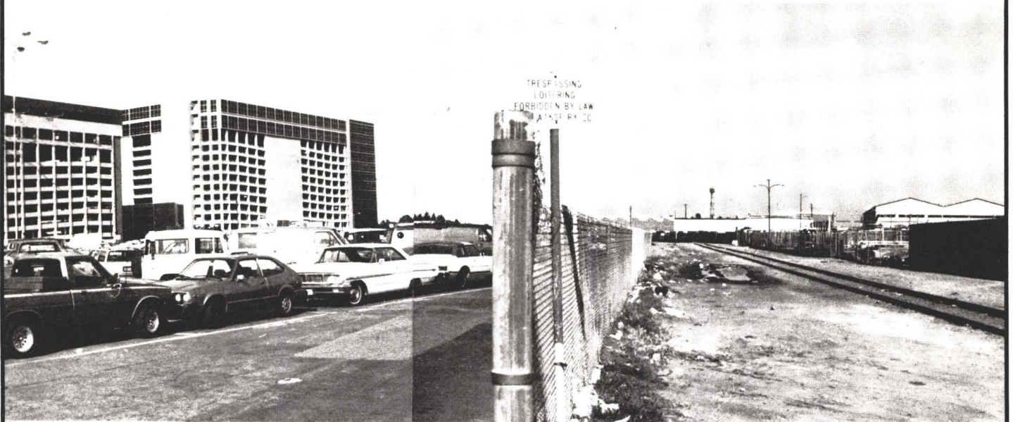
In the north, the rail line travels from Aviation Blvd. Station on an aerial structure above the existing Atchinson, Topeka and Santa Fe Railroad spur line. The top photo looks east from the intersection of Douglas Street and the railroad right-of-way. Buildings shown are Rockwell Corporation on the left of the photo and Northrop on the right. The lower photo shows the proximity of the proposed alignment to Kilroy Center and other major developments along Imperial Highway.
