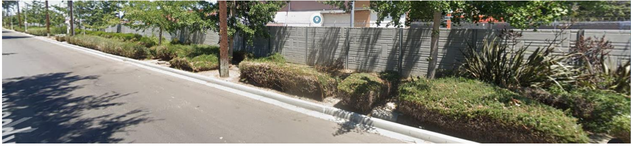
Figure 3.3-59. Examples of Existing Metro Soundwalls
