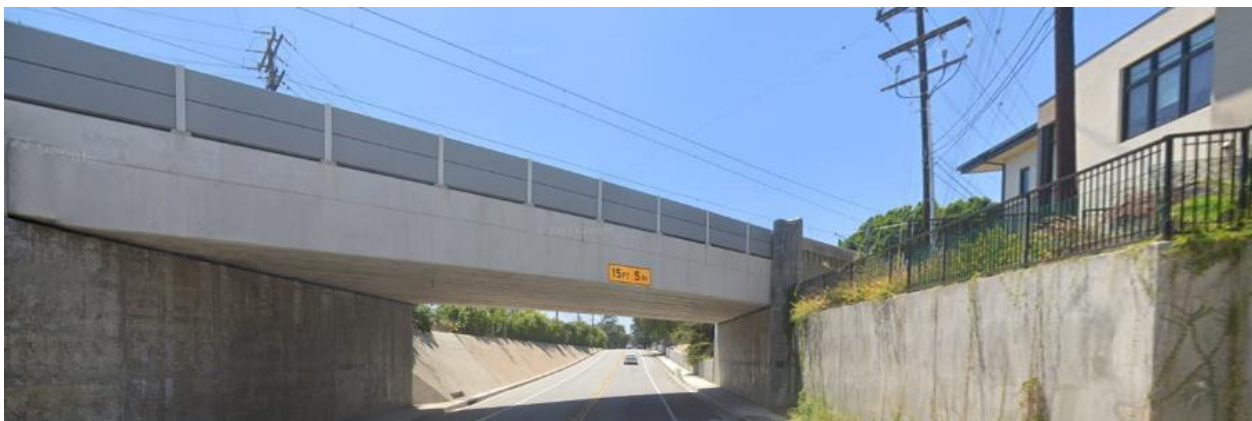
Above is one view of soundwalls on an elevated alignment of the existing Metro L Line (Gold).
