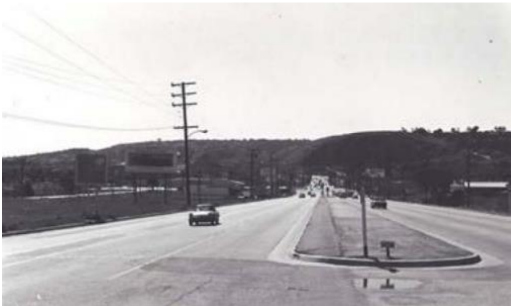
Figure 3.13-4. Hawthorne Boulevard following roadway redevelopment in 1960s
