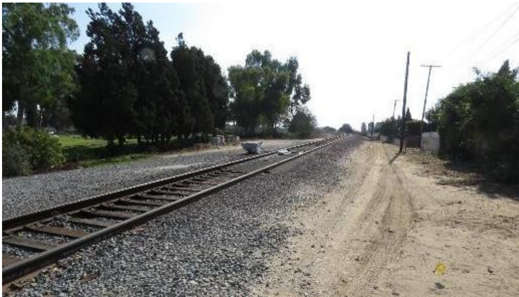
Figure 3.7-7. Metro ROW with current freight track, south of 182nd Street; facing south
