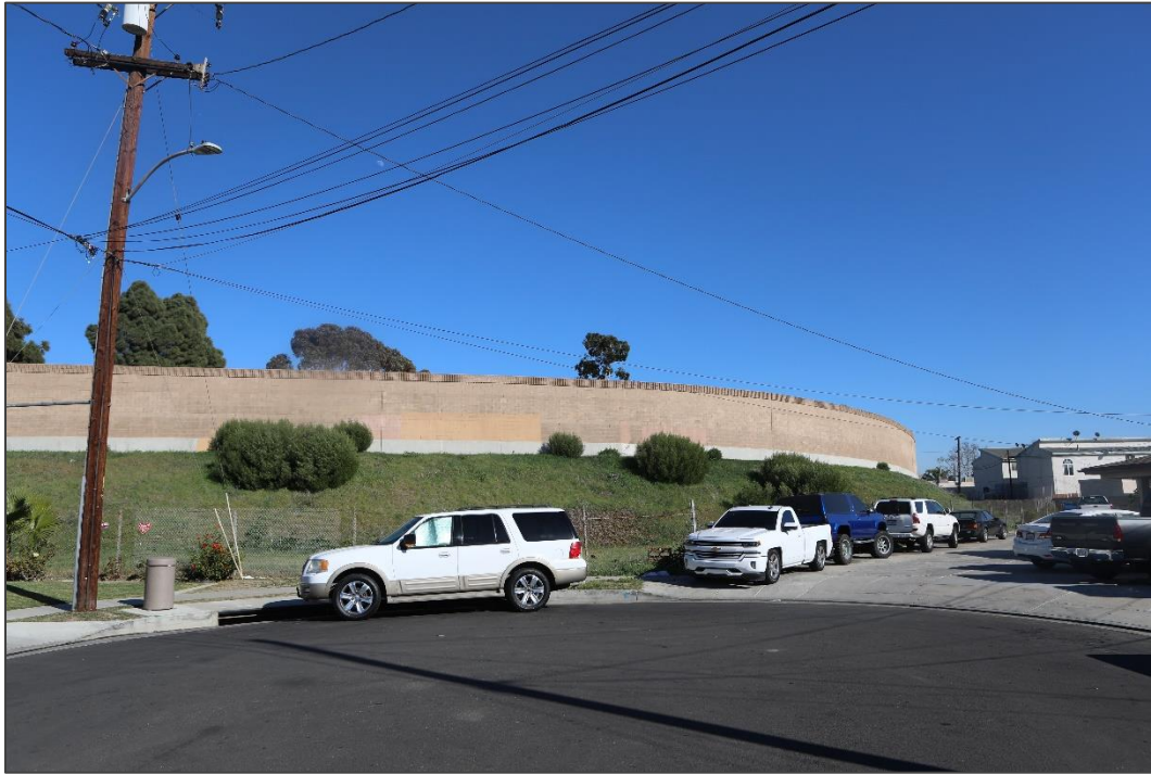
Figure 3.3-74. KOP 16 – Before and After Simulation View, View looking northeast from 161st Street towards the Hawthorne Option Elevated Alignment
