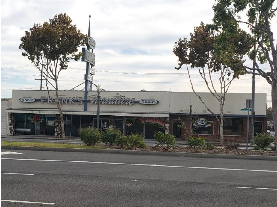
Figure 3.13-9. Overview of 16418-16424 Hawthorne Boulevard property, view to east, November 5, 2020
