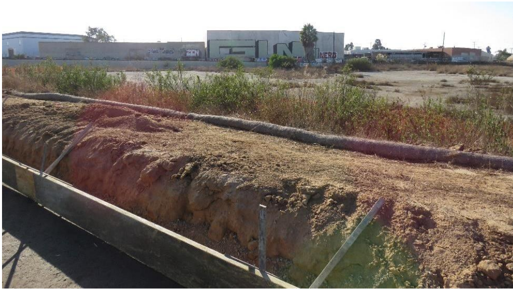
Figure 3.7-6. View Across Torrance TC Towards Proposed Station at Torrance TC; facing southwest
