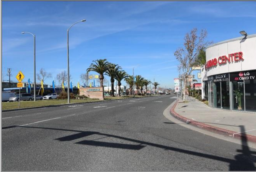
Figure 3.3-78. KOP 20 – Before and After Simulation View, View looking north/northwest from Hawthorne Boulevard towards the Hawthorne Option Elevated Alignment
