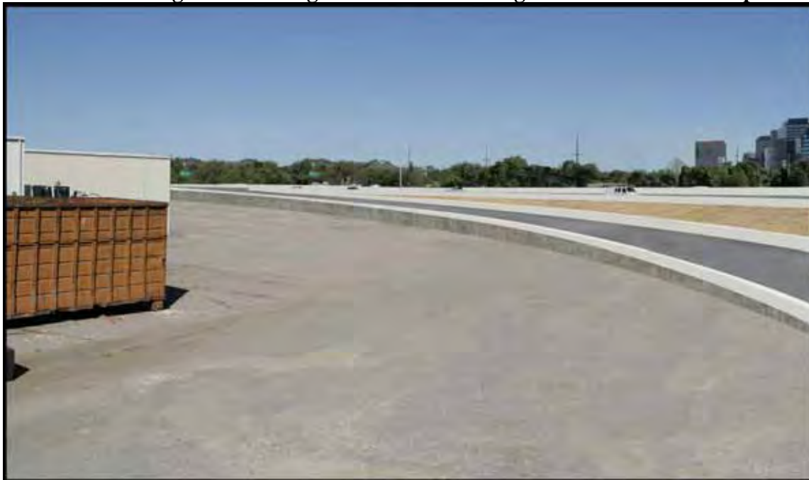
Figure 3.6-8: Viewpoint 2 (Proposed) – Veterans Administration Transportation Yard/Storage Area Facing East Towards Realigned S/B I-405 Off-ramp
