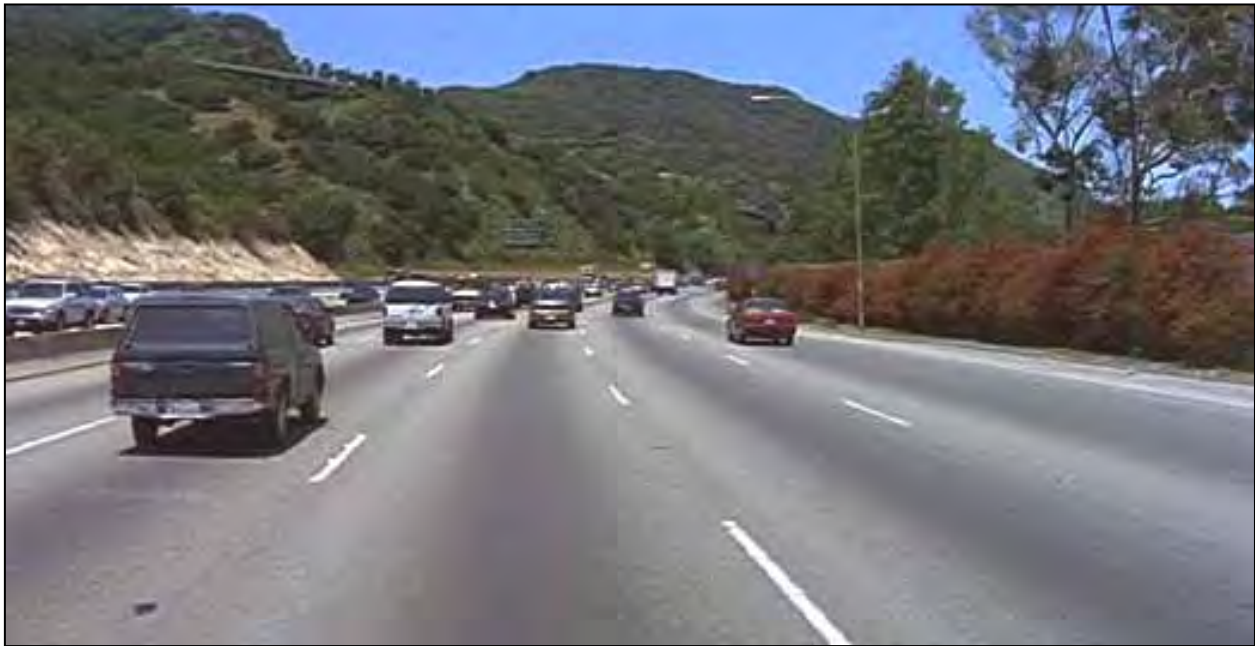
Figure 3.6-11: Viewpoint 4 (Existing) – Northbound I-405 Towards Getty Center Drive
