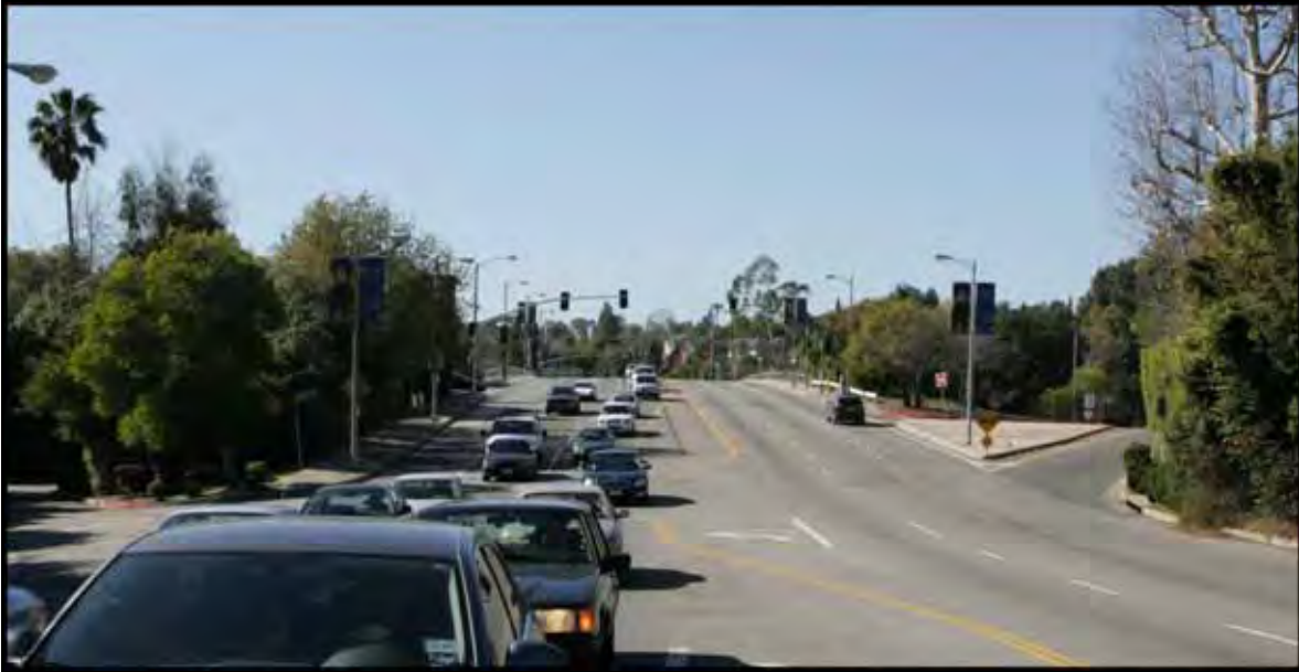
Figure 3.6-9: Viewpoint 3 (Existing) – Sunset Blvd. Overcrossing Facing West
