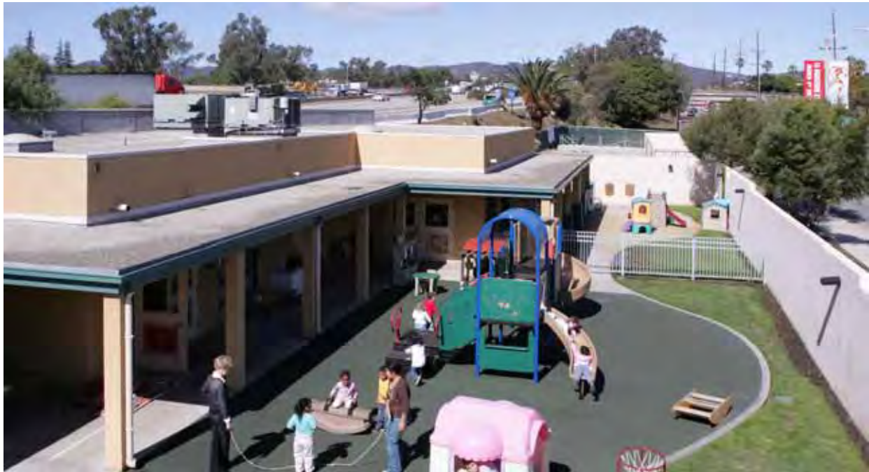
Figure 3.6-3: Viewpoint 1 (Existing) – The Salvation Army Westwood Transitional Village and Bessie Pregerson Child Development Center
