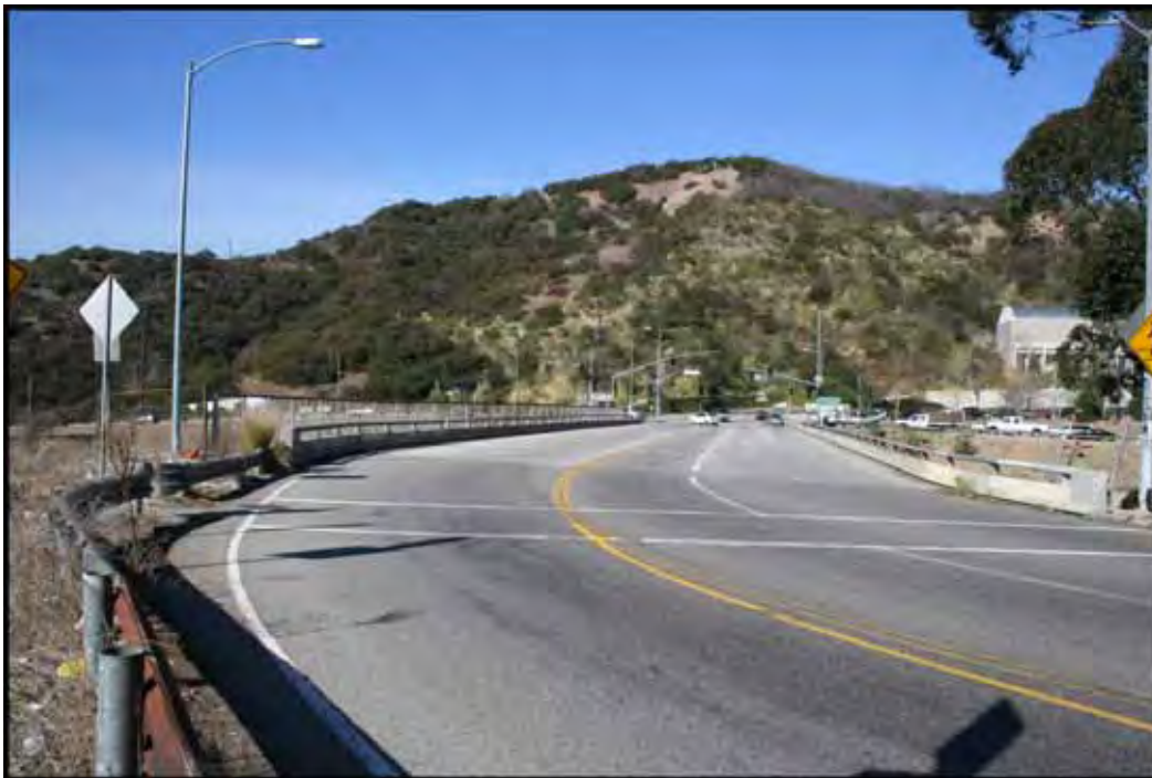
Figure 3.6-13: Viewpoint 5 (Existing) – Skirball Center Drive Overcrossing Facing West
