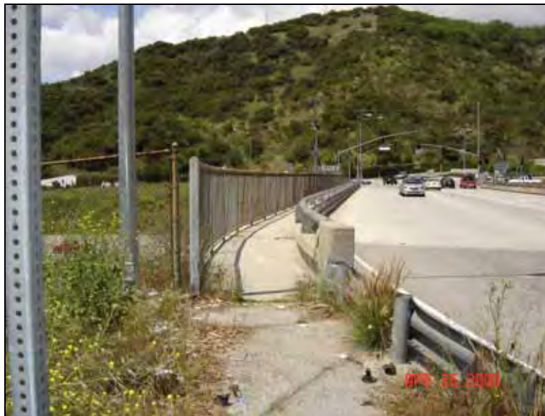
Figure 3.17-4: Skirball Center Drive Overpass (Looking West)
