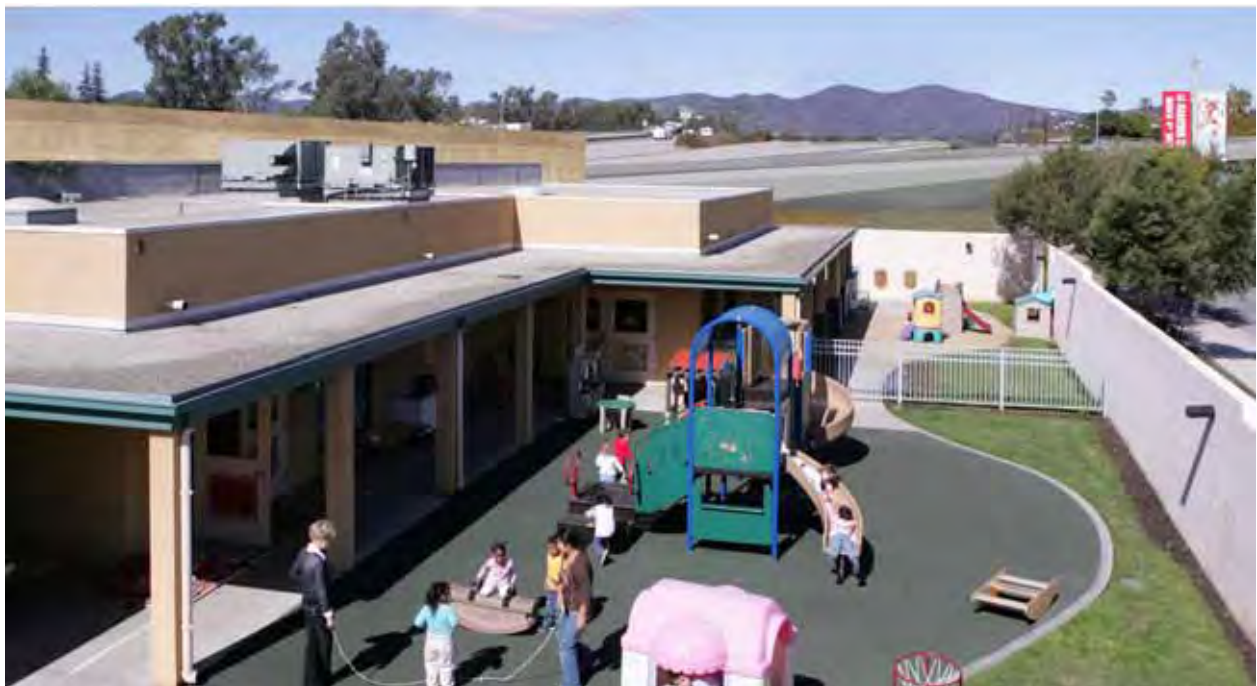
Figure 3.6-4: Viewpoint 1 (Proposed) – The Salvation Army Westwood Transitional Village and Bessie Pregerson Child Development Center with Proposed Soundwall
