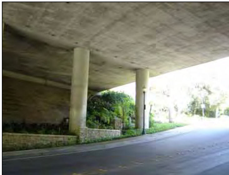
Figure 3.17-3: Columns and Embankment Underneath I-405 at Bel Air Crest Road
