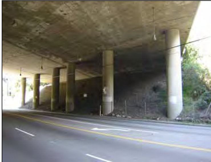
Figure 3.17-2: Columns and Embankments Underneath I-405 at Sepulveda Blvd.
