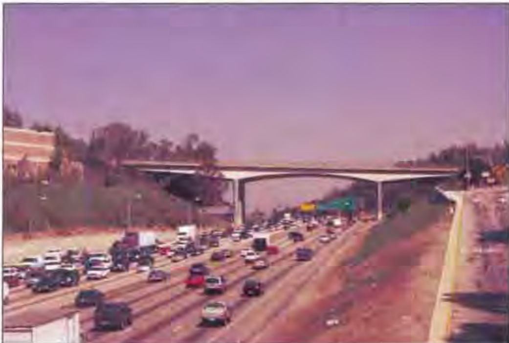
Figure 7: Mulholland Drive Overcrossing
