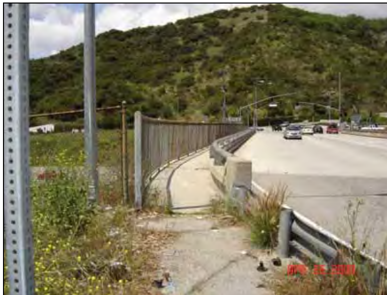
Figure 3.17-4: Skirball Center Drive Overpass (Looking West)
