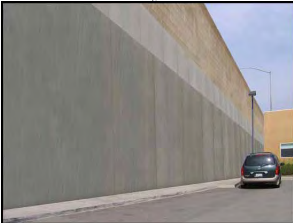
Figure 3.6-5: Viewpoint 3 (Proposed) – The Salvation Army Westwood Transitional Village and Bessie Pregerson Child Development Center Parking Lot with Proposed Soundwall Atop a Retaining Wall
