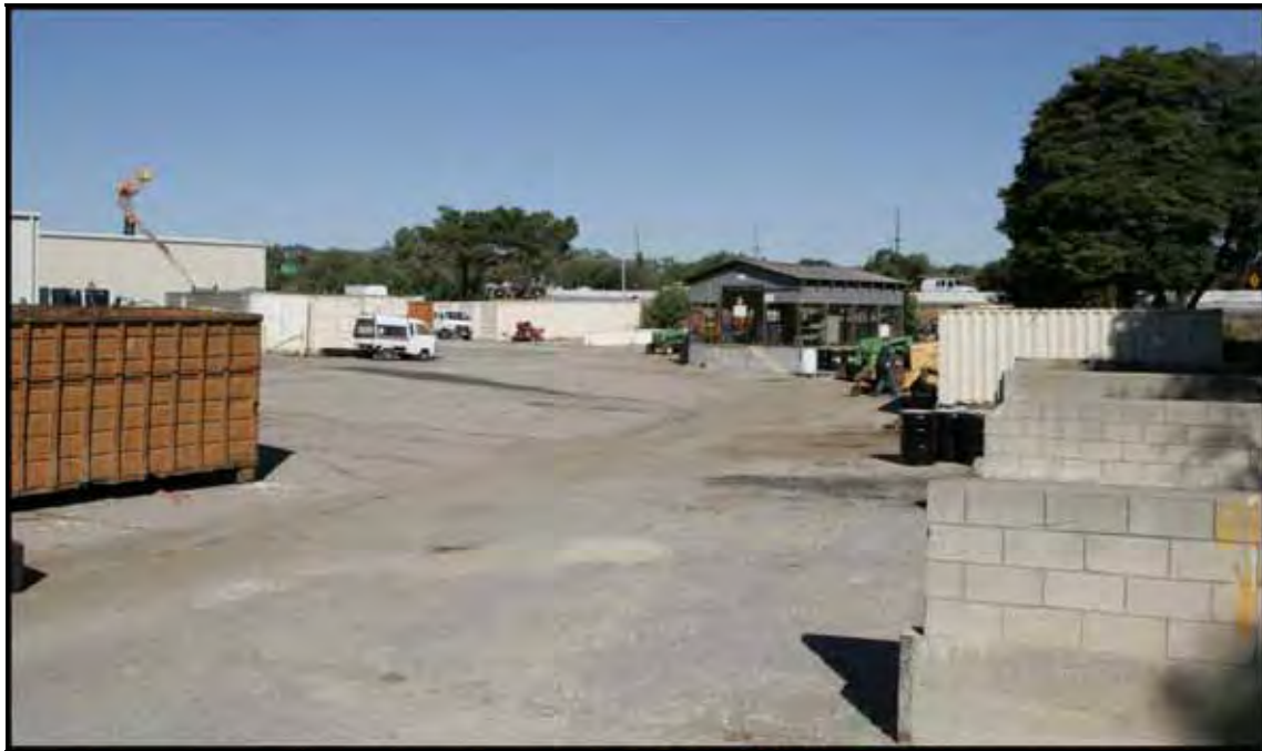
Figure 3.6-8: Viewpoint 5 (Existing) – Veterans Administration Center’s Storage Area Facing East Towards S/B I-405
