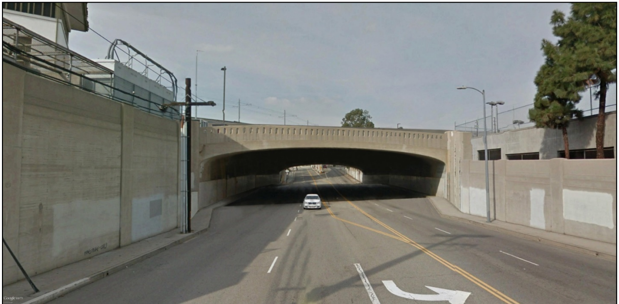
Figure 8-9. Key View #2a – Vignes Street Bridge (view looking west toward bridge) Post-Project Conditions
