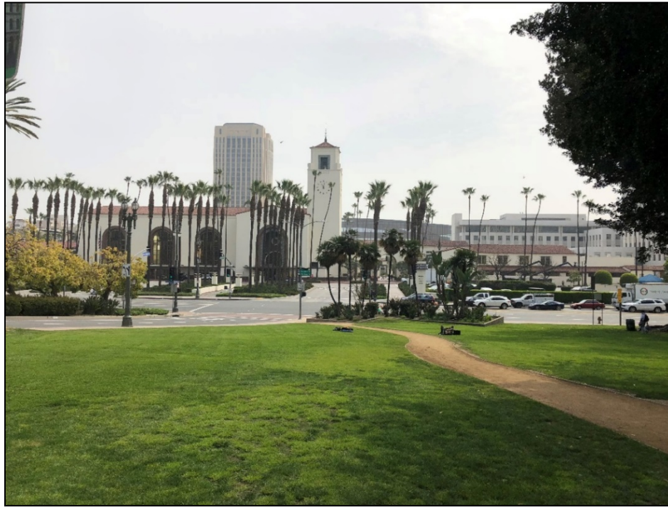
Figure 8-19. Key View #4b – Los Angeles Union Station Entrance (view looking east from Father Serra Park toward Los Angeles Union Station) Post-Project Conditions
