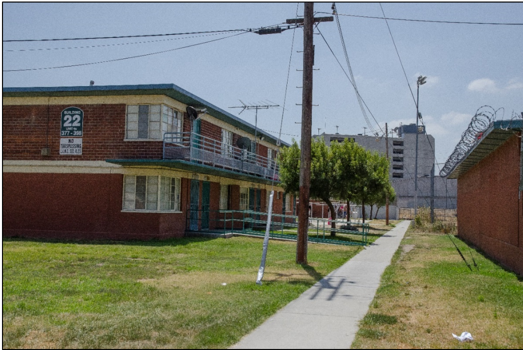
Figure 8-6. Key View #1b – Existing Conditions
