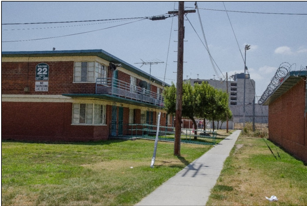
Figure 8-4. Key View #1b – Existing Conditions
