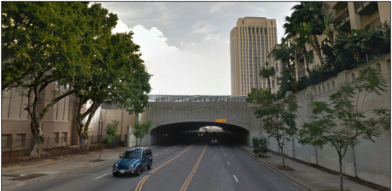
Figure 8-15. Key View #3b – Cesar Chavez Avenue Bridge (view looking east toward bridge) Post-Project Conditions
