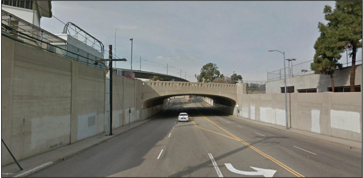
Figure 8-8. Key View #2a – Vignes Street Bridge (view looking west toward bridge) Existing Conditions
