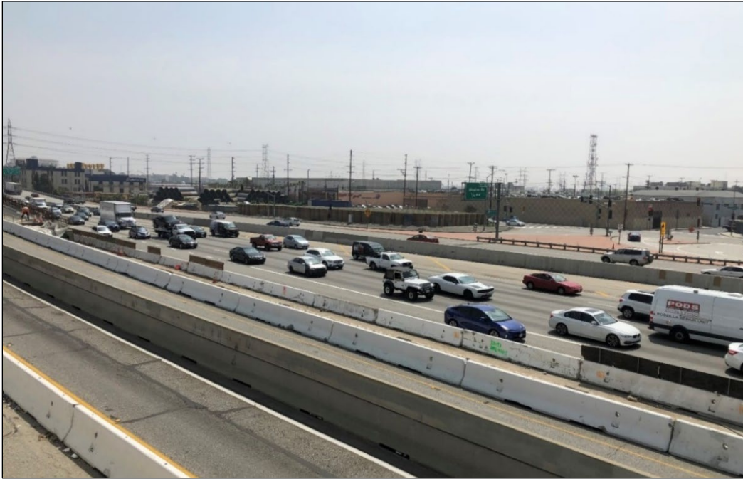
Figure 4-10. Key View #5a - US-101/Commercial Street (view looking southeast from Los Angeles Union Station southern platform limit toward US-101/Commercial Street)
