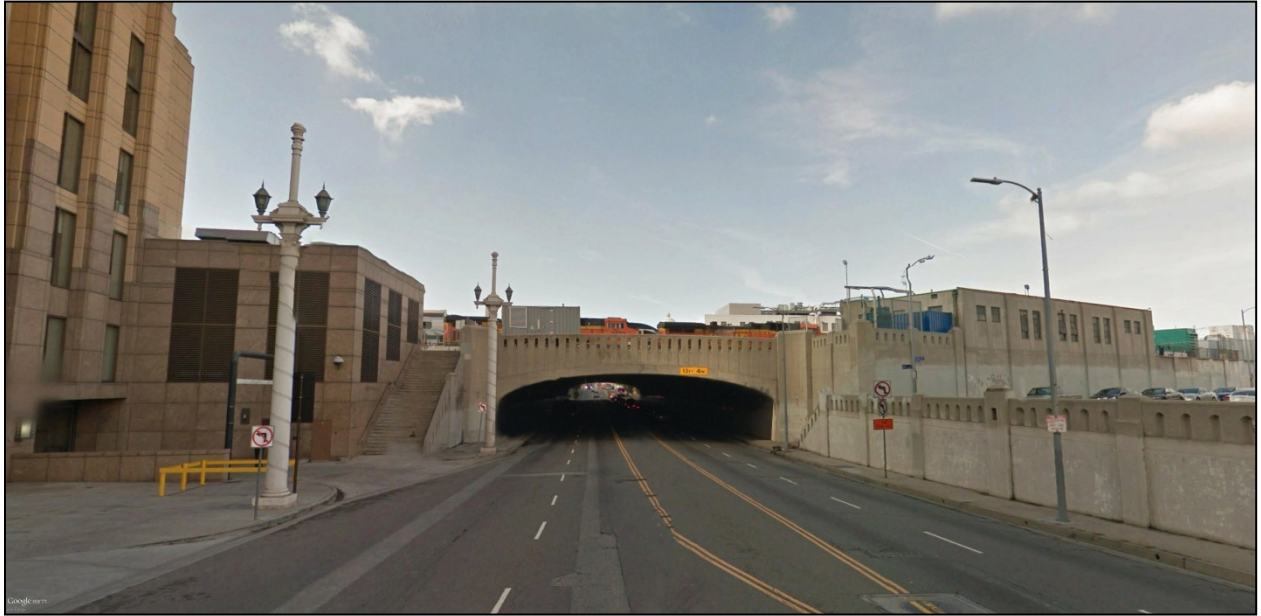
Figure 8-12. Key View #3a – Cesar Chavez Avenue (view looking west toward bridge) Existing Conditions
