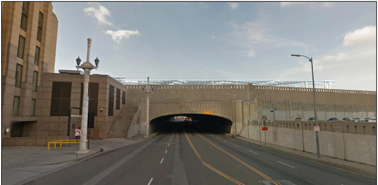
Figure 8-13. Key View #3a – Cesar Chavez Avenue (view looking west toward bridge) Post-Project Conditions
